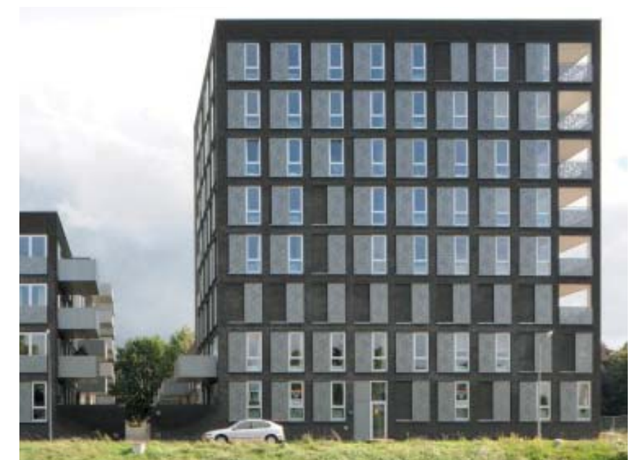
Beekport Housing Block, Maccreanor Lavington Architects Brick grid with vertical window in-fills and sliding shutters
