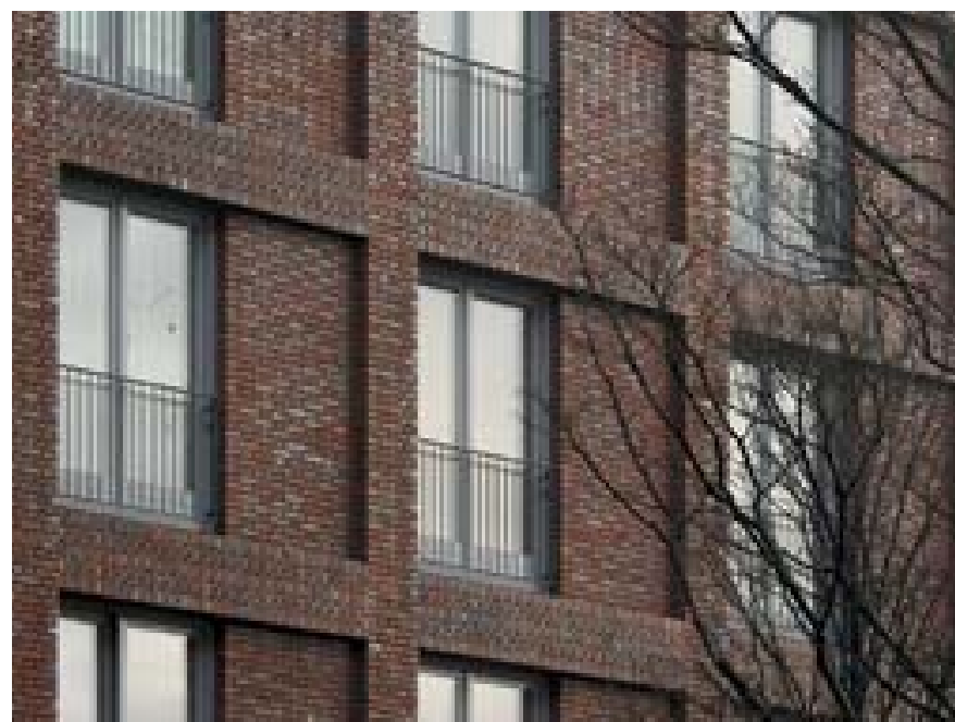
Oranjeleen Student Housing, Den Haag, Rapp & Rapp Architects Brick grid and set-back infill panels with vertical windows
