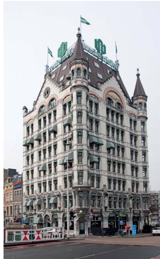
White House, Rotterdam 10 storey building articulated as a tower through vertical corner bays and three-storey mansard roof
