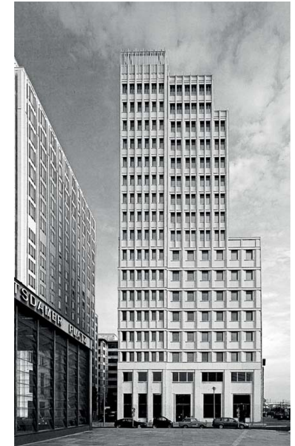
Dellbrueck-Haus, Berlin Architects: Hans Kollhoff 17/18 storey building, which reads as both a tower with slim vertical elements (left-hand- side) and a building (right-hand-side)
