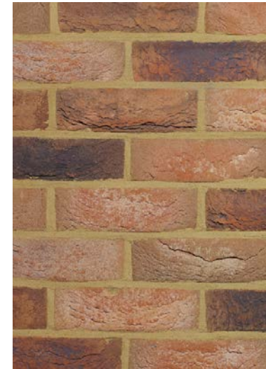
2. Wienerberger Heritage Blend Residential and workspace buildings
