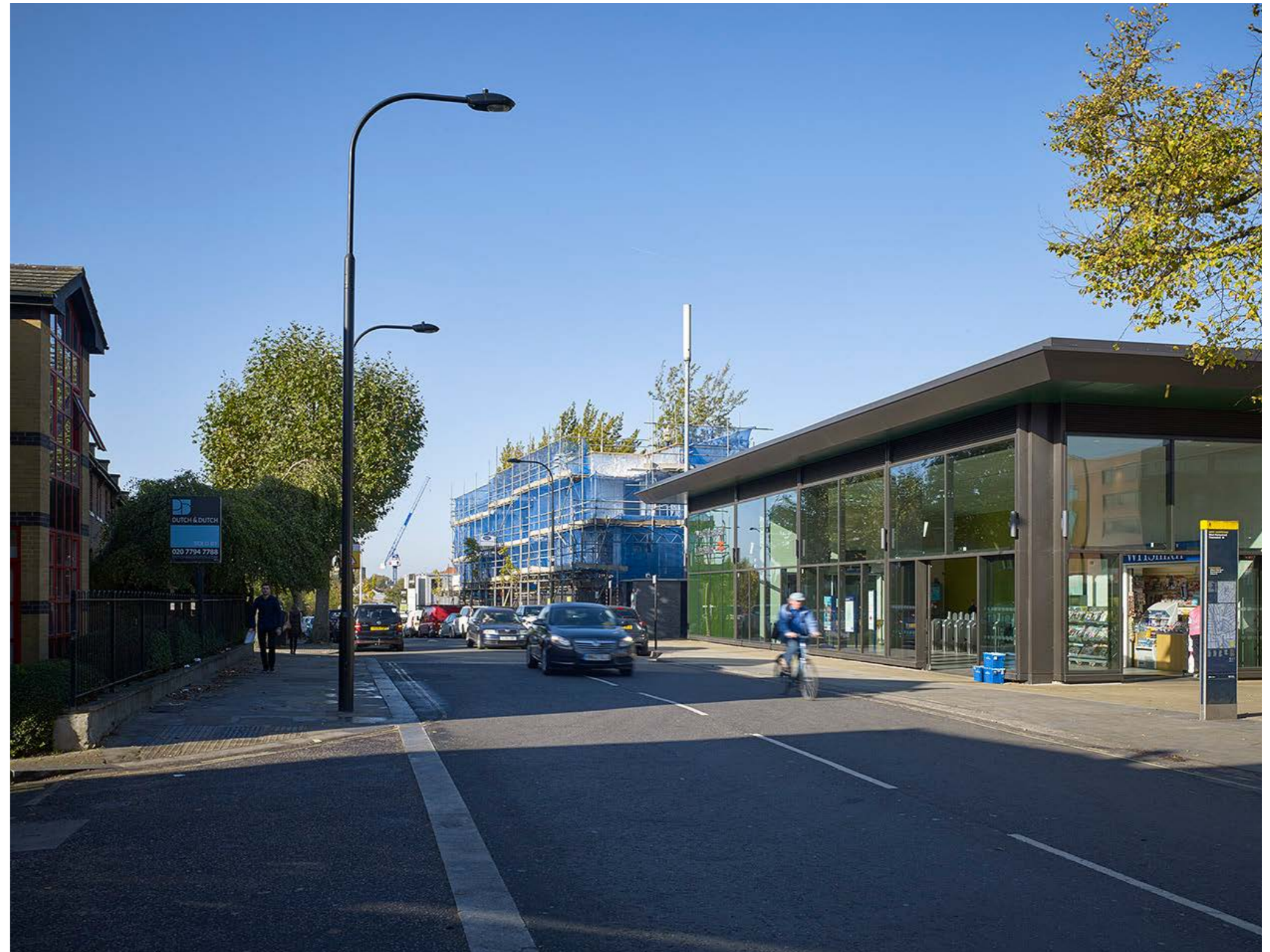
View 3 - Iverson Road looking west towards site
