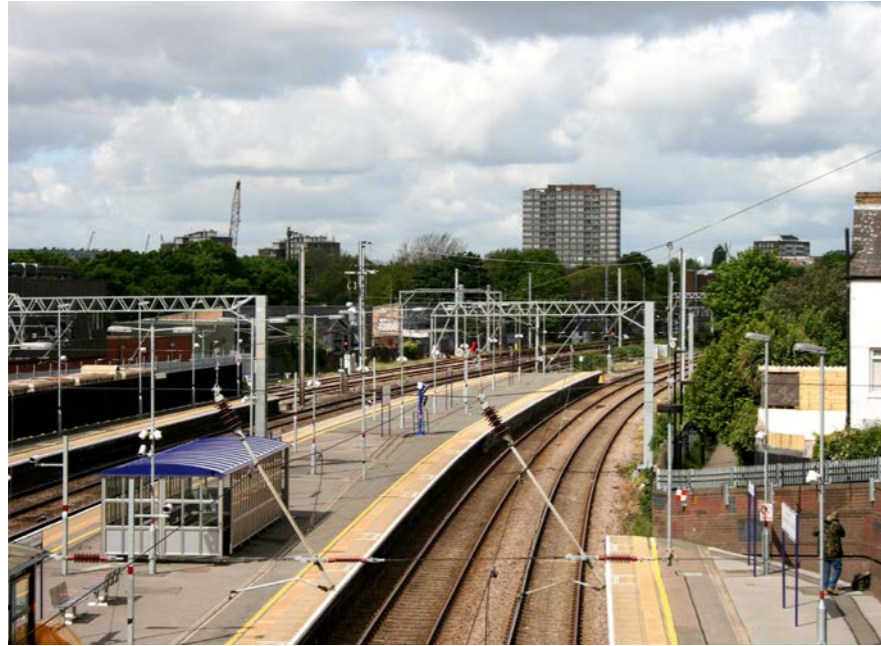
View from footbridge at West Hamsstead Thameslink station
