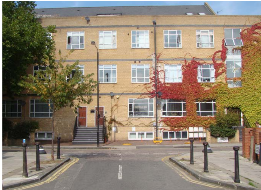
Existing workspace buildings in Maygrove Road
