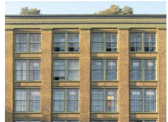
Five storey warehouse building, St John's Square, Clerkenwell
