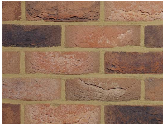
Light red, multi-textured stock brick in stretcher bond, Heritage Blend by Wienerberger or similar approved
