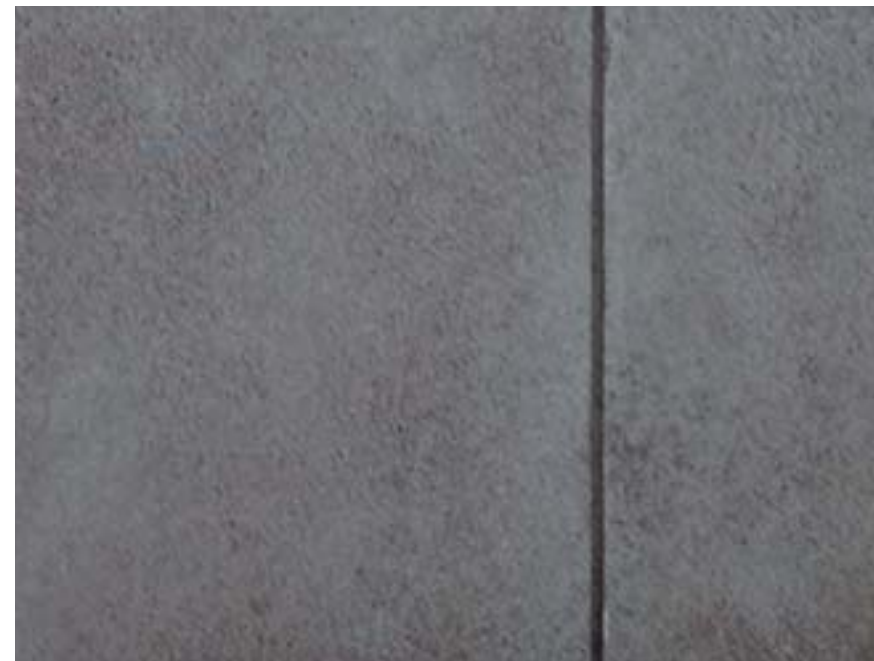
Red-tint Pre-Cast Concrete Reconstituted Stonework
