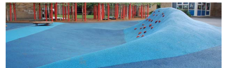
Porous wetpour soft play surface
