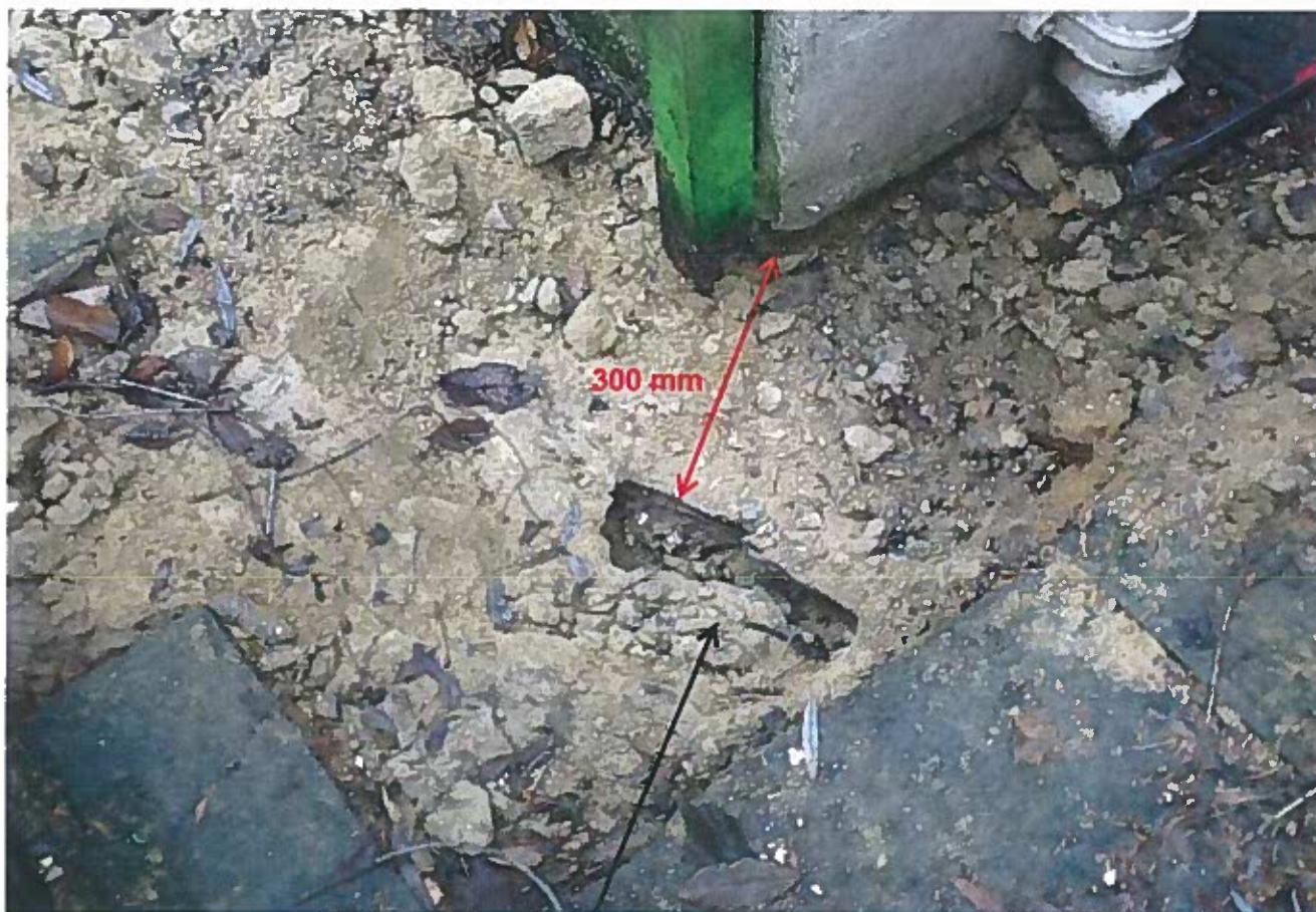
150 mm diameter pipe, set in concrete 100 mm below surface
