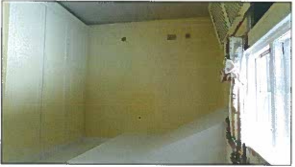
Wall H (attic floor)
