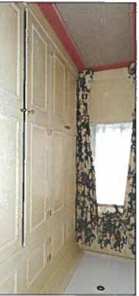
Existing photographs Wall G (second floor)
