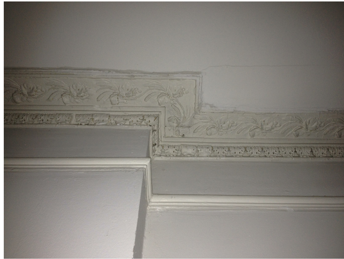
Existing CG-01 profile in Ground Floor Living Room
