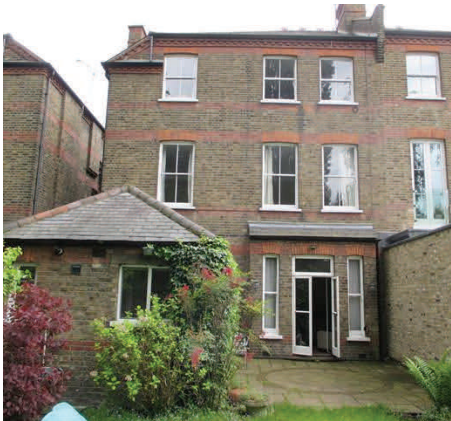
Existing rear façade of No. 23 Downside Crescent
