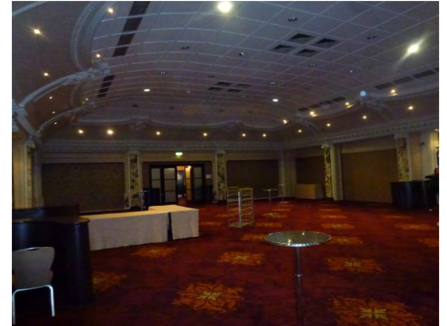
Figure 30: View of the Woburn Suite, showing the relatively plain wall and ceiling insertions between its historic plasterwork. The area of ceiling tiles in the centre of the ceiling represents the former location of its glass roof.
