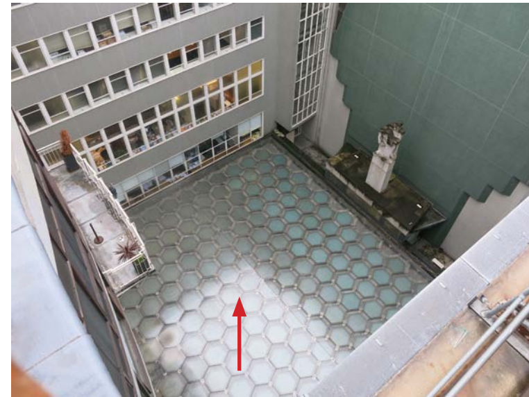
3 Secondary rainscreen glazing destroys the integrity of original roof below and leaks through perished mastic joints
