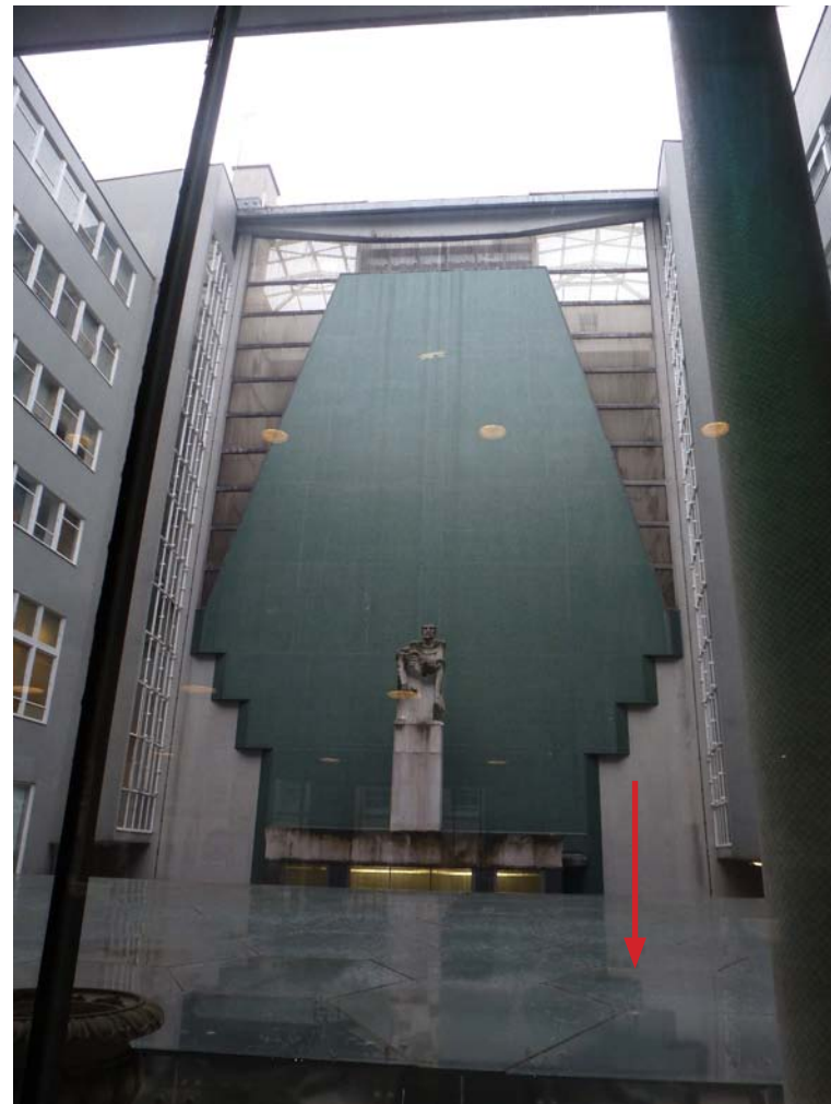
5 Dust settles on secondary rainscreen and is hard to clean without damaging roof resulting in reduced transparency
