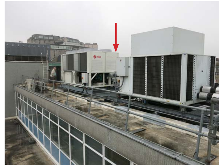
3 Existing rooftop plant chillers and associated pipework to be retained
