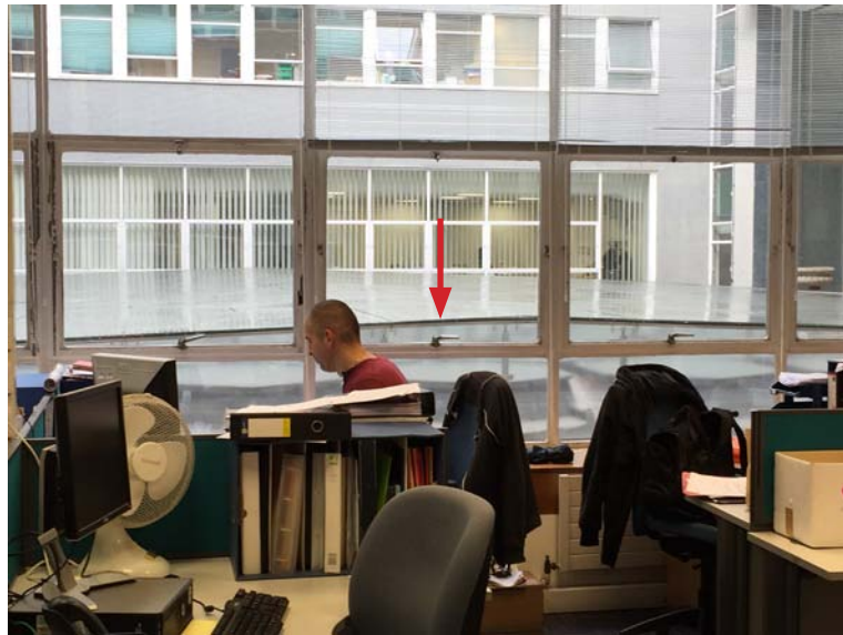
1 Secondary rainscreen glazing visually encroaches on office space reducing outlook
