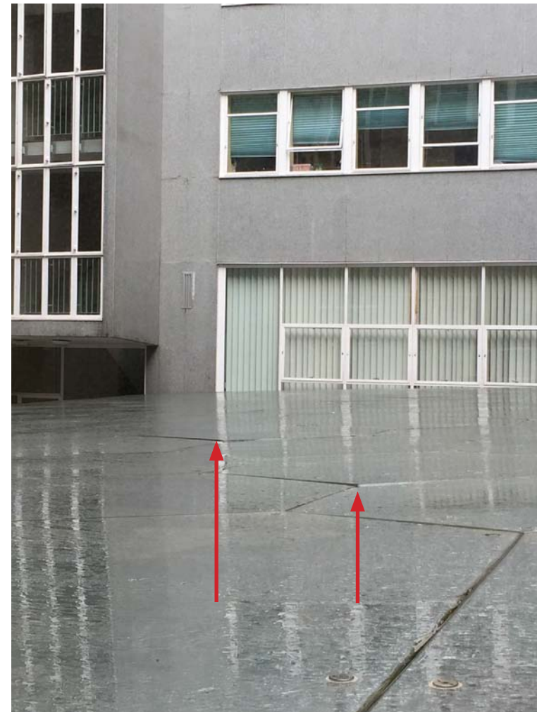
6 Secondary rainscreen glazing has become disjointed permitting pooled water to leak through perished mastic joints
