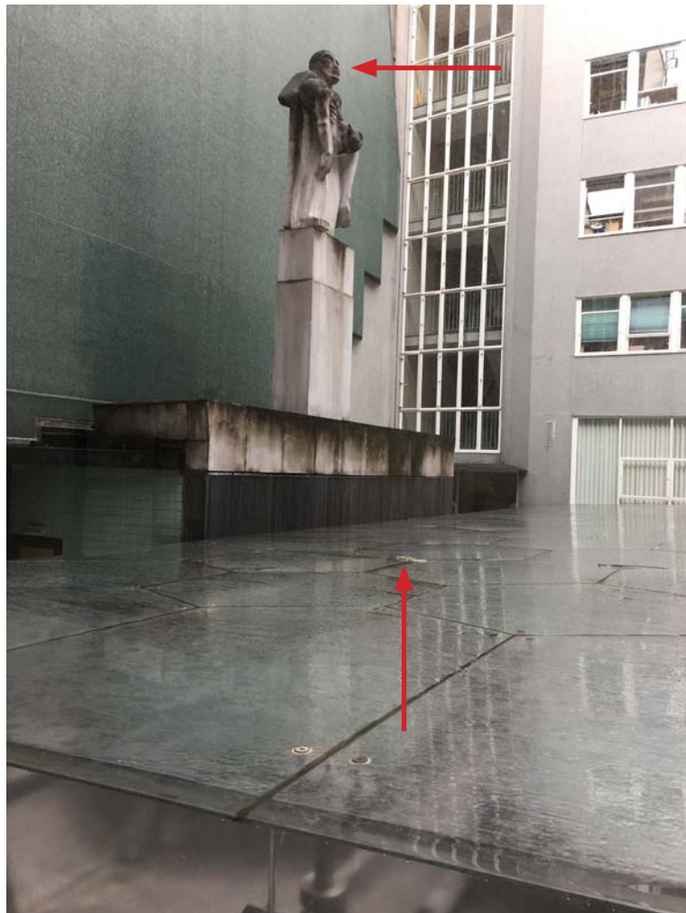
4 Perished mastic joints in secondary rainscreen glazing are impossible to rectify without destroying visual integrity. Sir Jacob Epstein's 'Pieta' sculpture is stained black due to constant exposure to the elements
