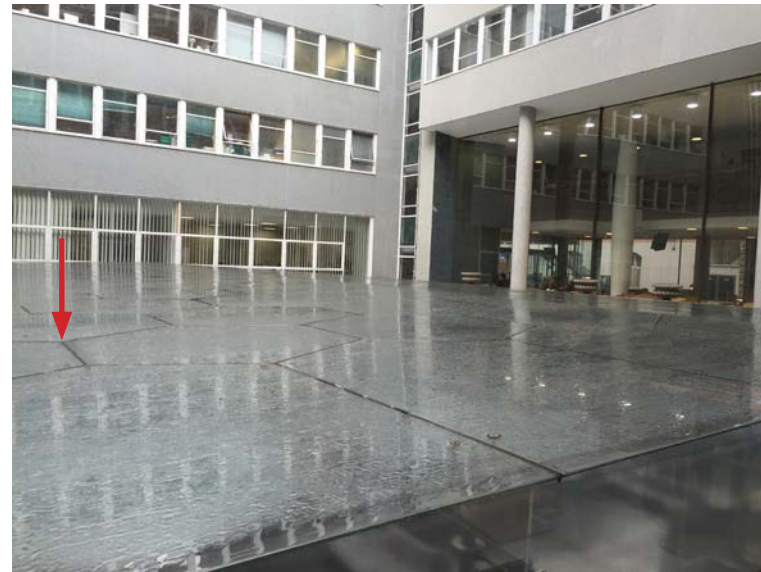
2 Secondary rainscreen glazing has become disjointed permitting pooled water to leak through perished mastic joints
