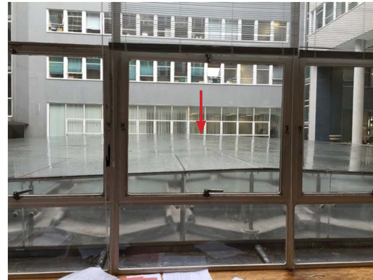
3 Secondary rainscreen glazing reduces interconnectivity between windows either side of courtyard
