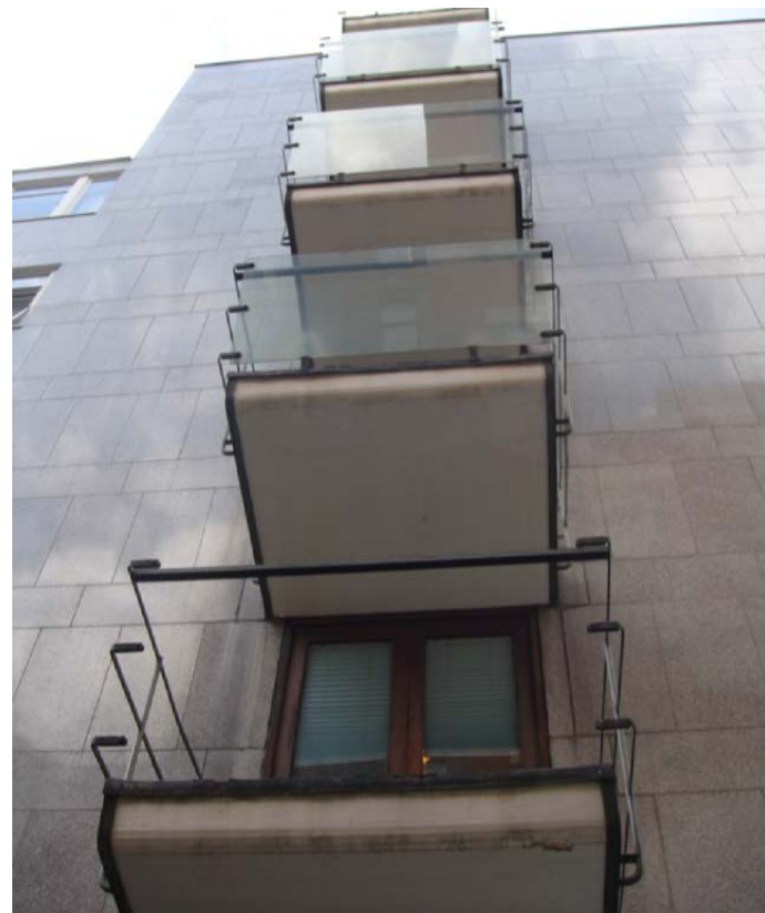
Recent view showing 1st floor balcony with missing glass panel. Subsequently the remaining glass was removed for safety
