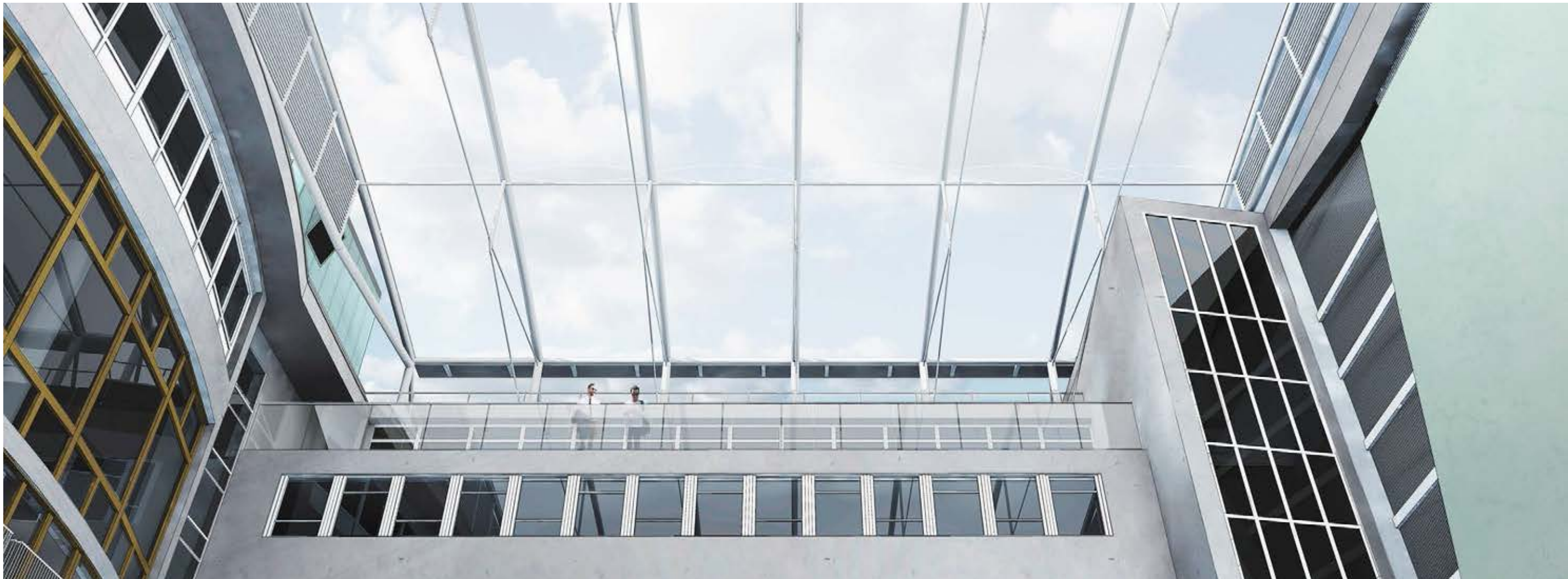
This submission proposes the installation of a gently curving ETFE roof spanning from north to south. The scheme allows reinstatement of the original roof over the conference hall and could also allow refurbishment of sixth floor balconies and removal of the black metal mesh on the west elevation of the Council Chamber, partially restoring its original transparency.
