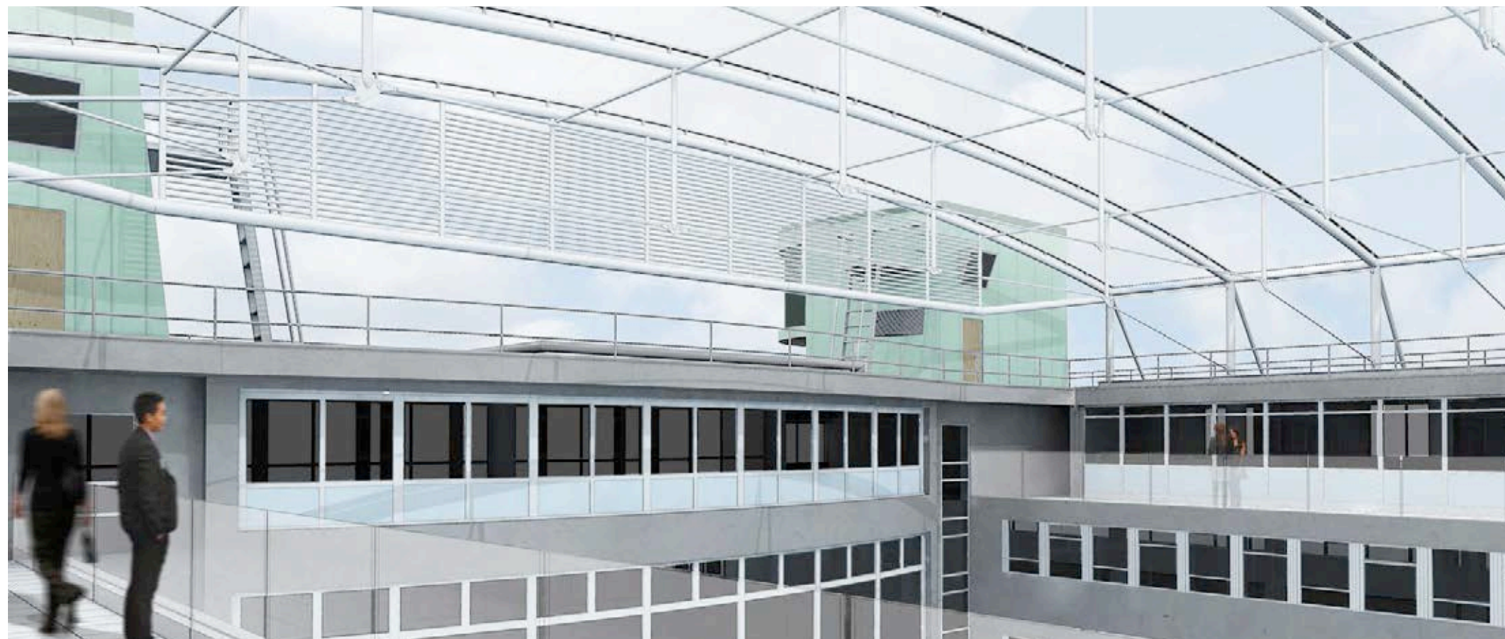
Proposed view across the courtyard from the refurbished 6th floor balconies. The louvred screen helps to break up wind driven rain. Note also removal of black metal mesh from Council Chamber glazing (bottom left)
