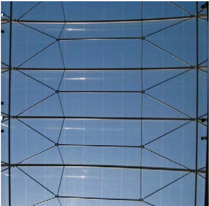
Looking up at the ETFE and steel at Devonshire Square
