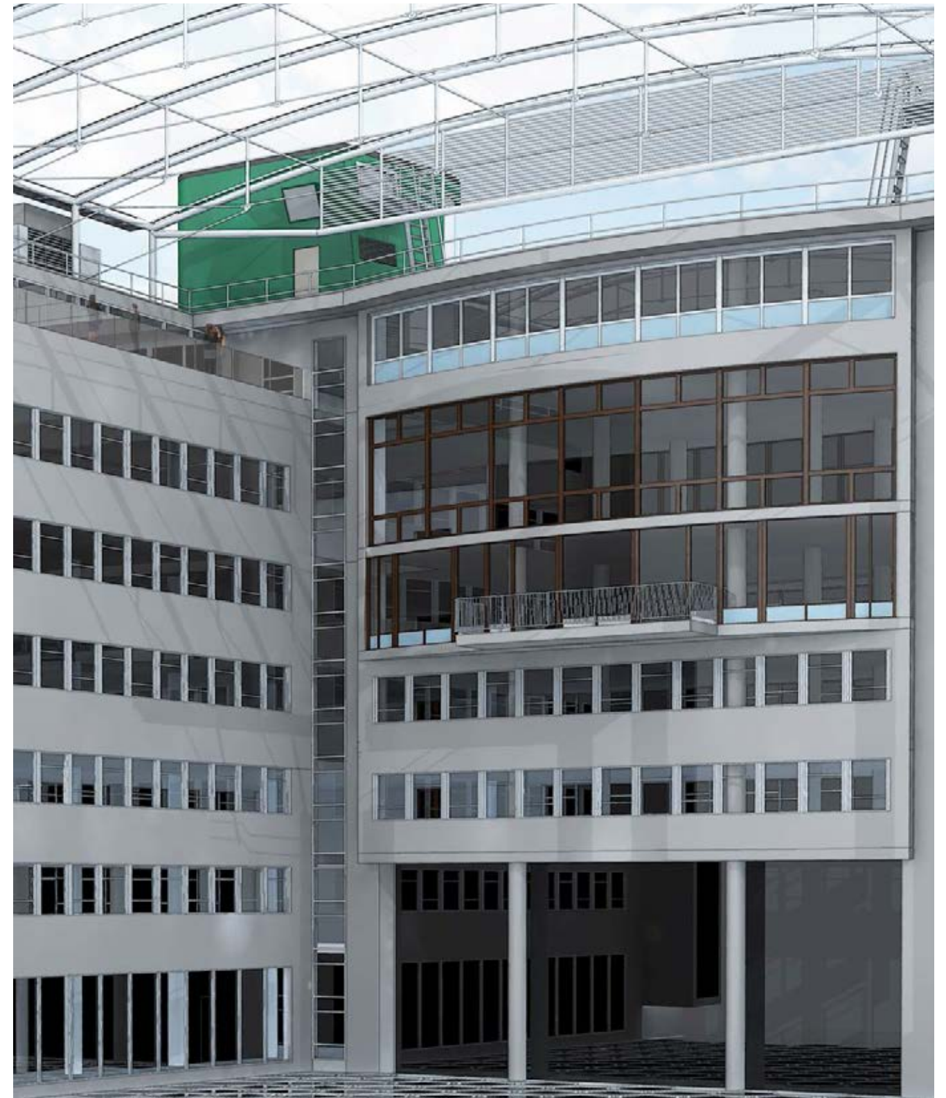
The glass over-cladding is removed and the courtyard is protected by a gently curving ETFE roof with minimal lightweight steel structure. The view of the original roof from the Marble Hall is restored. Note also the removal of black metal mesh from Council Chamber glazing.
