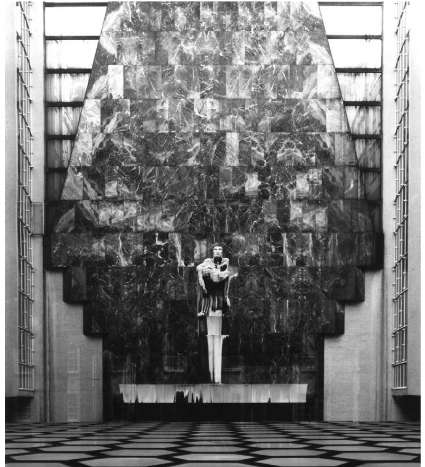
View from the Marble Hall across the Conference Hall roof (1958). The marble cladding to the Memorial Wall was replaced with mosaic after fixings for the marble failed.
