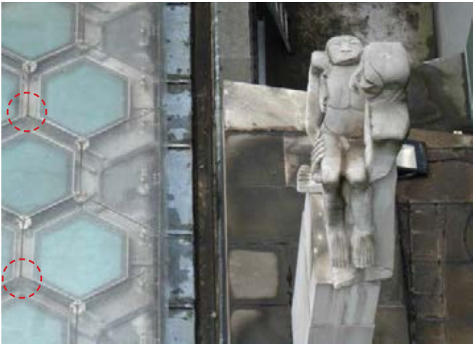
Detail view. Note missing stanchions to some corners of overcladding
