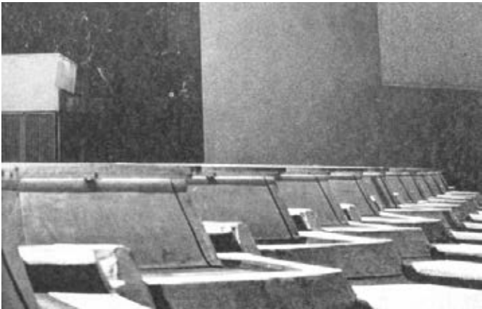
Detail view of rooflight kerbs (1957)
