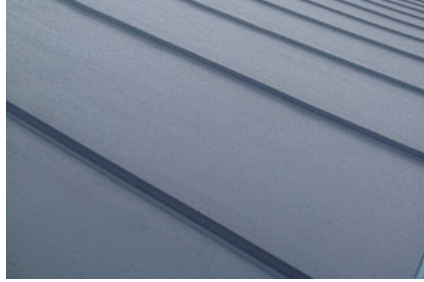
grey roofing material
