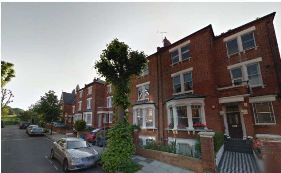
Front elevation of 62 Parliament Hill and rest of the terrace
