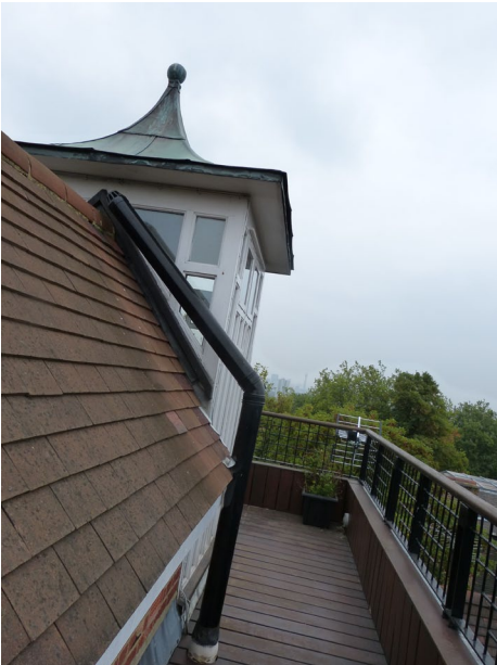
Existing boiler flue
