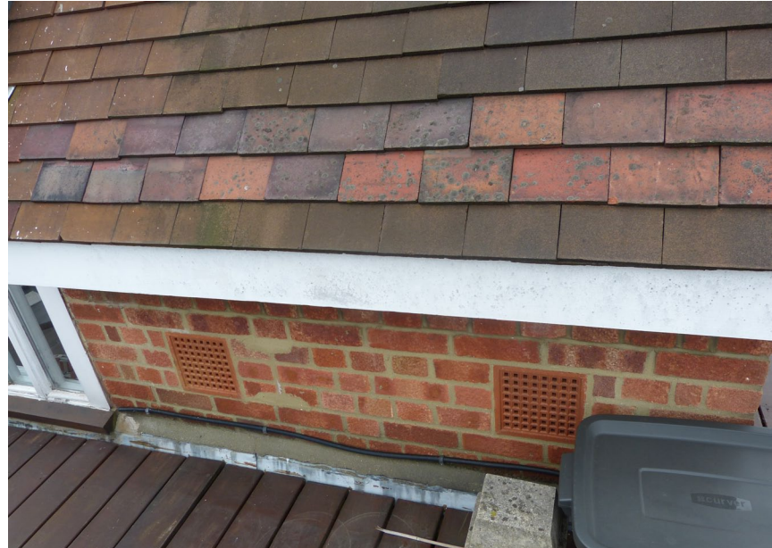
Overhang of pitched roof to lift overrun
