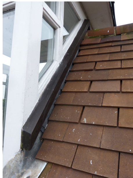
Poor detailing between the two structures
