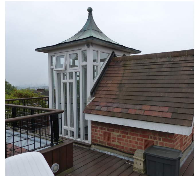
Photo showing the glazed timber conservatory providing access via a narrow spiral stair with a copper roof and also the brick lift over run with the pitched red clay roof.
