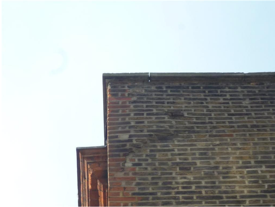
PHOTOGRAPH 11: Defective parapet brickwork to south east corner.
