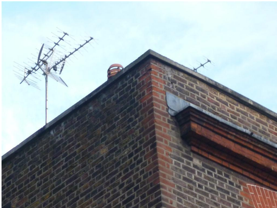
PHOTOGRAPH 12: Isolated spalled bricks to south west corner – to be replaced.
