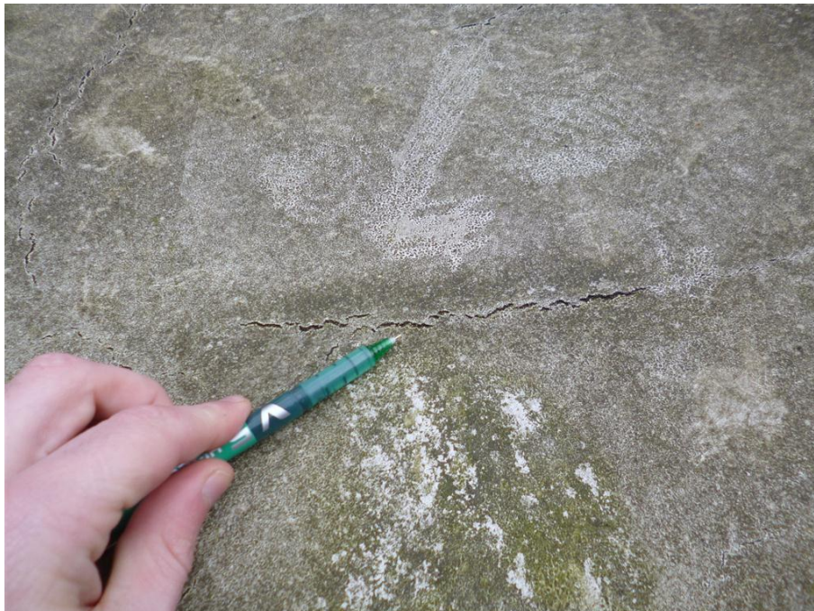
PHOTOGRAPH 10: Typical cracking to lantern light roofs – poultice repairs proposed.
