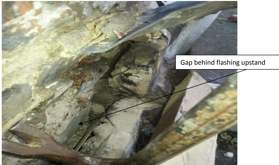
Plate 2: Section showing a horizontal gap at the base of wall behind timber wall plate and flashing upstand.
