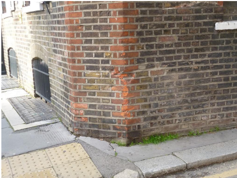
PHOTOGRAPH 8: Impact damaged brickwork.
