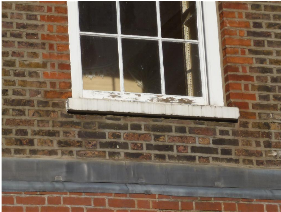
PHOTOGRAPH 7: Poor decorations to sash windows.
