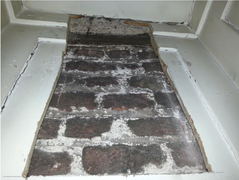
Plate 4: Reveal of the brickwork details behind the timber panelling in the approx location of the external cracking of the gable wall.
