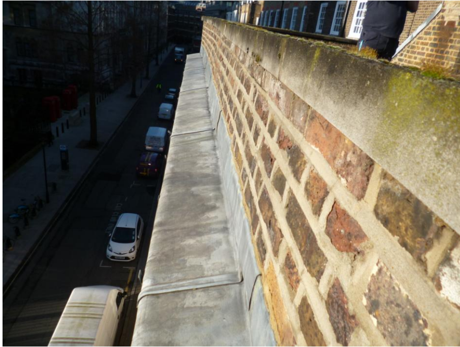
PHOTOGRAPH 3: Movement of front Carey Street parapet wall.
