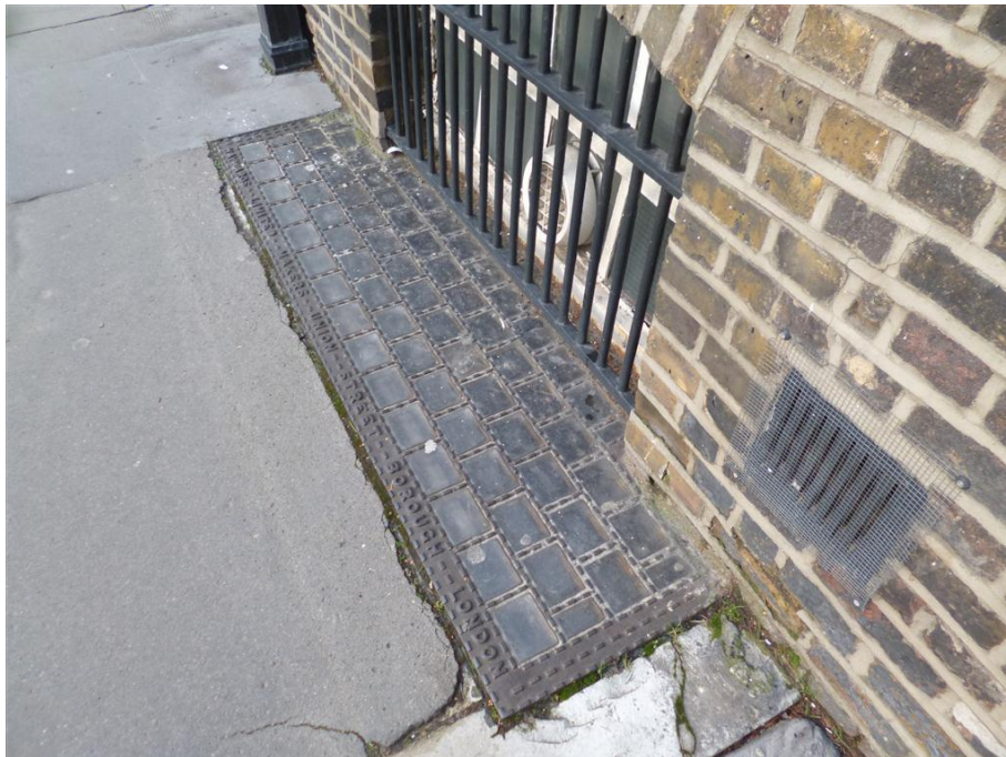
PHOTOGRAPH 4: Typical pavement light externally.
