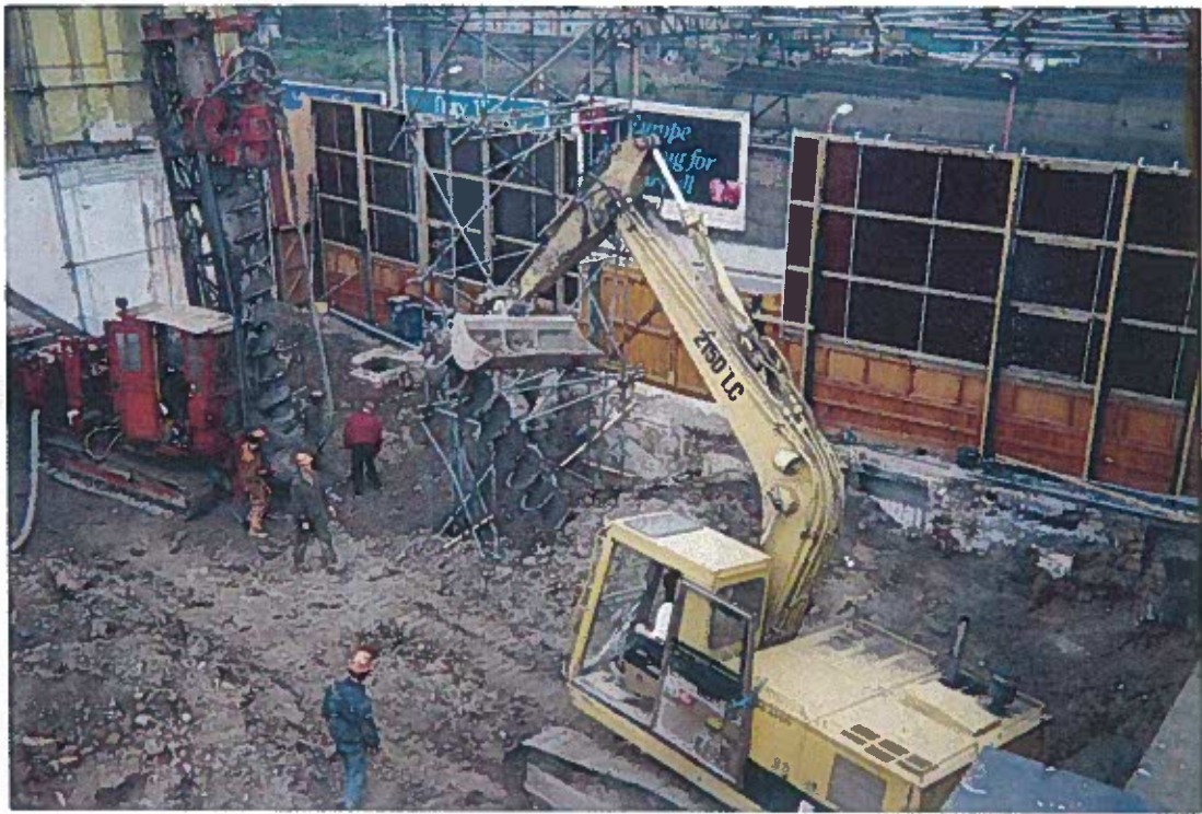
[Wonder Construction] 258 Belsize Road London NW6
