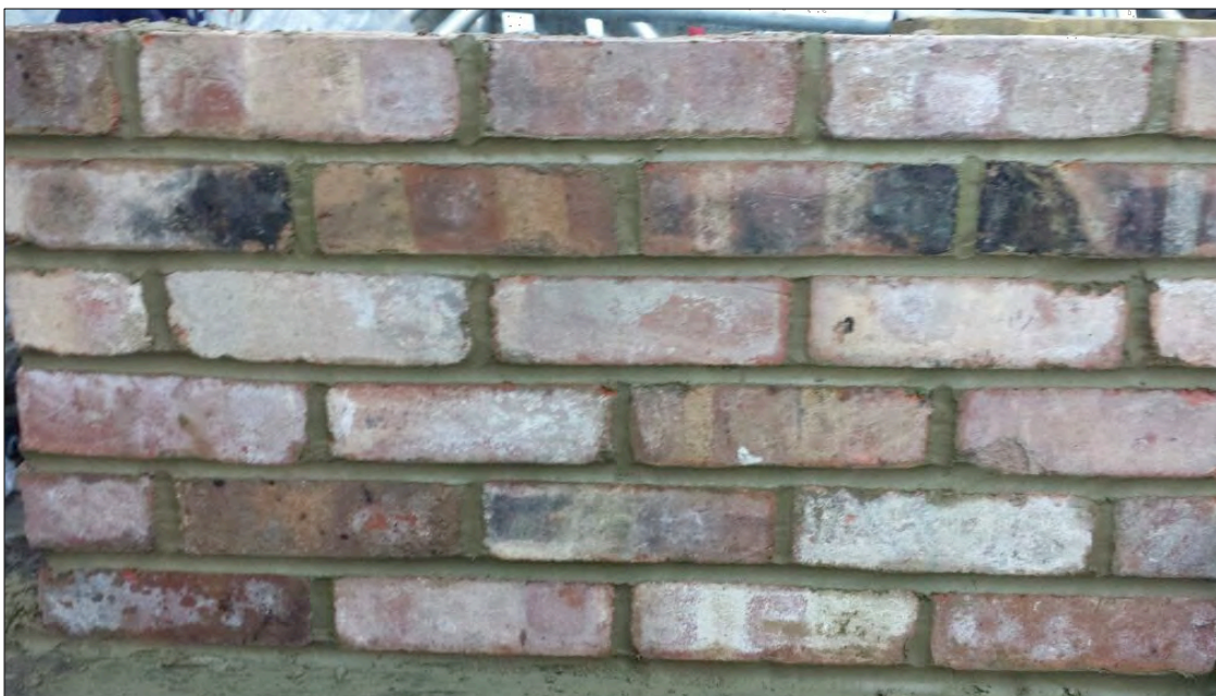
2 Revised Facing Brick Sample Panel Photo 2 N.T.S.
