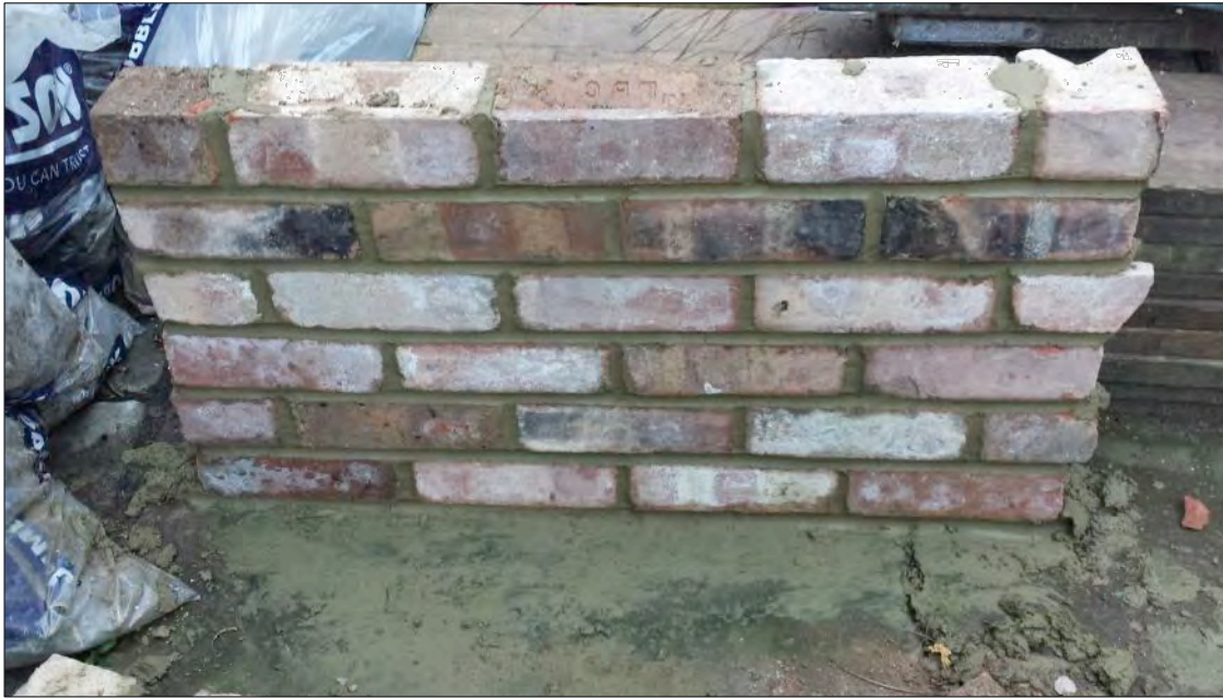
1 Revised Facing Brick Sample Panel Photo 1 N.T.S.
