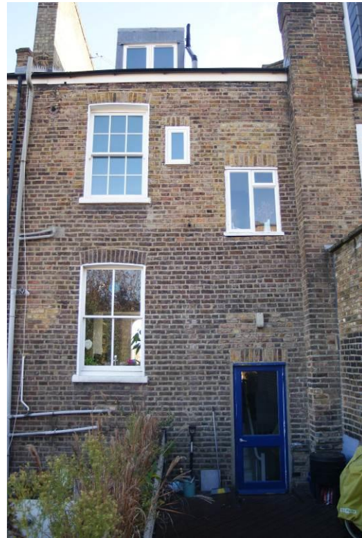
09. 119B Queens Crescent, Existing Rear Elevation from Roof Terrace
