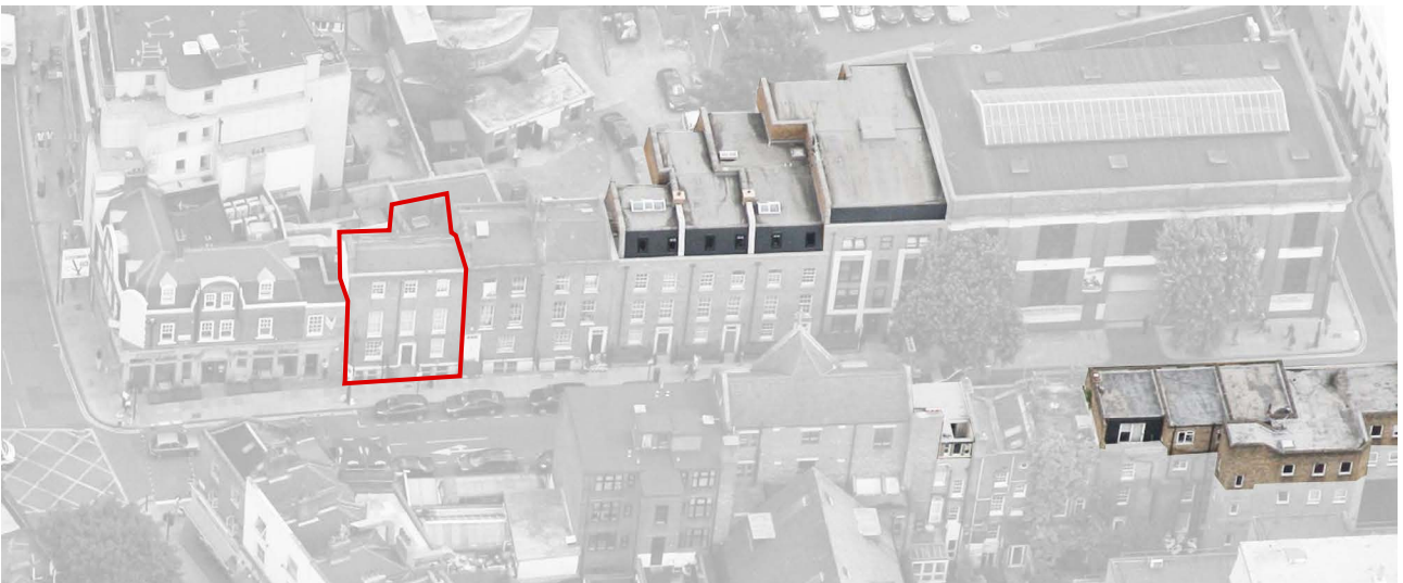
02. Consented Planning Schemes for rooftop developments on Arlington Road.
