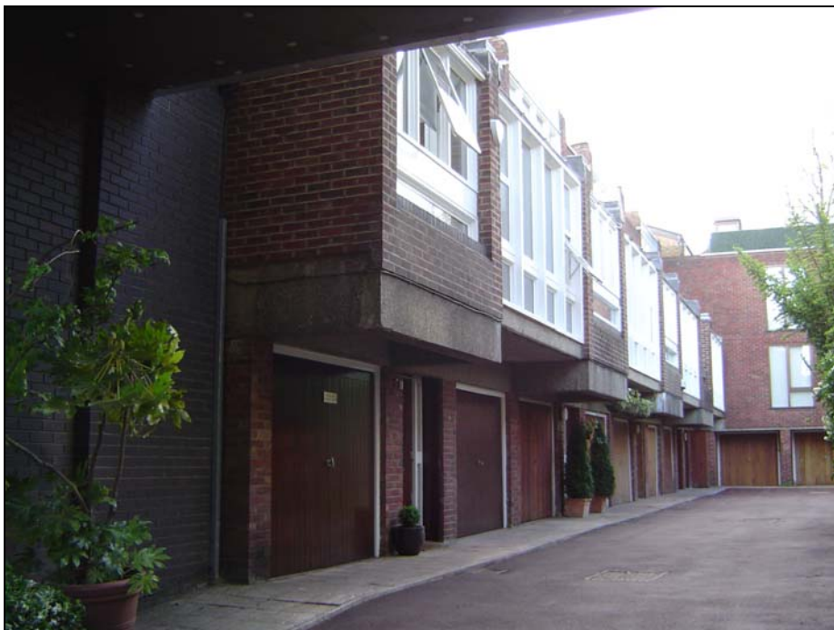
Plate D : Looking down Lakis Close towards the neighbouring property
