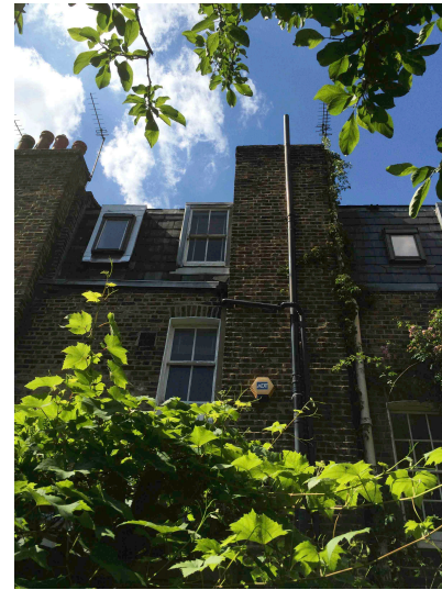
REAR ELEVATION - UPPER from garden
