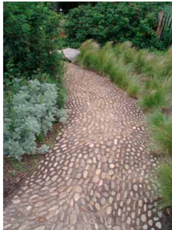
Boulders and natural river stones set into concrete mortar bed - larger stones / slabs transitioning to cobbles and pebbles.
