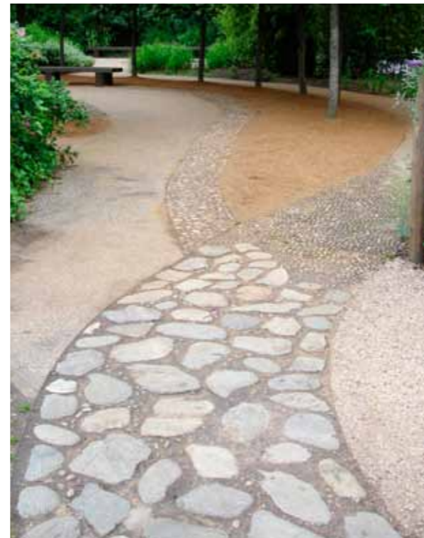
Boulders and natural river stones set into concrete mortar bed - larger stones / slabs transitioning to cobbles and pebbles.
