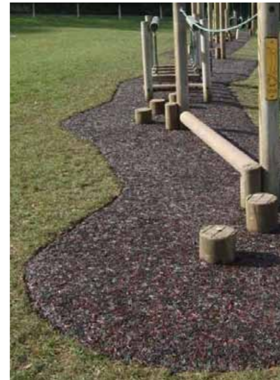
Rubber Safety Surface: Recycled tyre chippings simulating natural bark, laid on existing ground.
