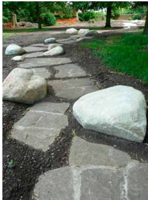
Boulders and natural river stones set into concrete mortar bed - larger stones / slabs transitioning to cobbles and pebbles.
