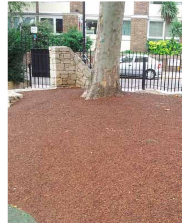
Rubber Safety Surface: Recycled tyre chippings simulating natural bark, laid on existing ground.
