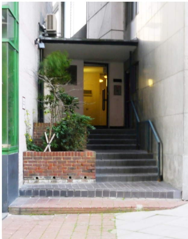
Centre Heights residential entrance at Belsize Road
