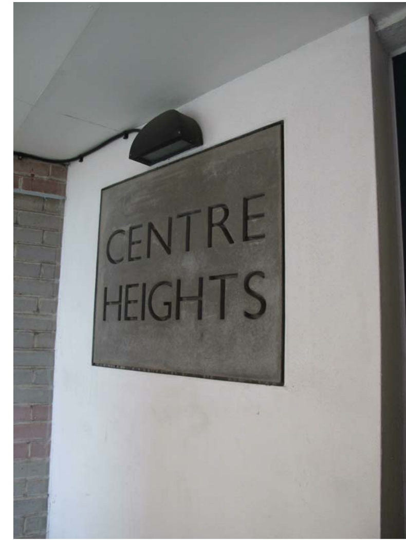
4 Existing concrete sign and downlighting
