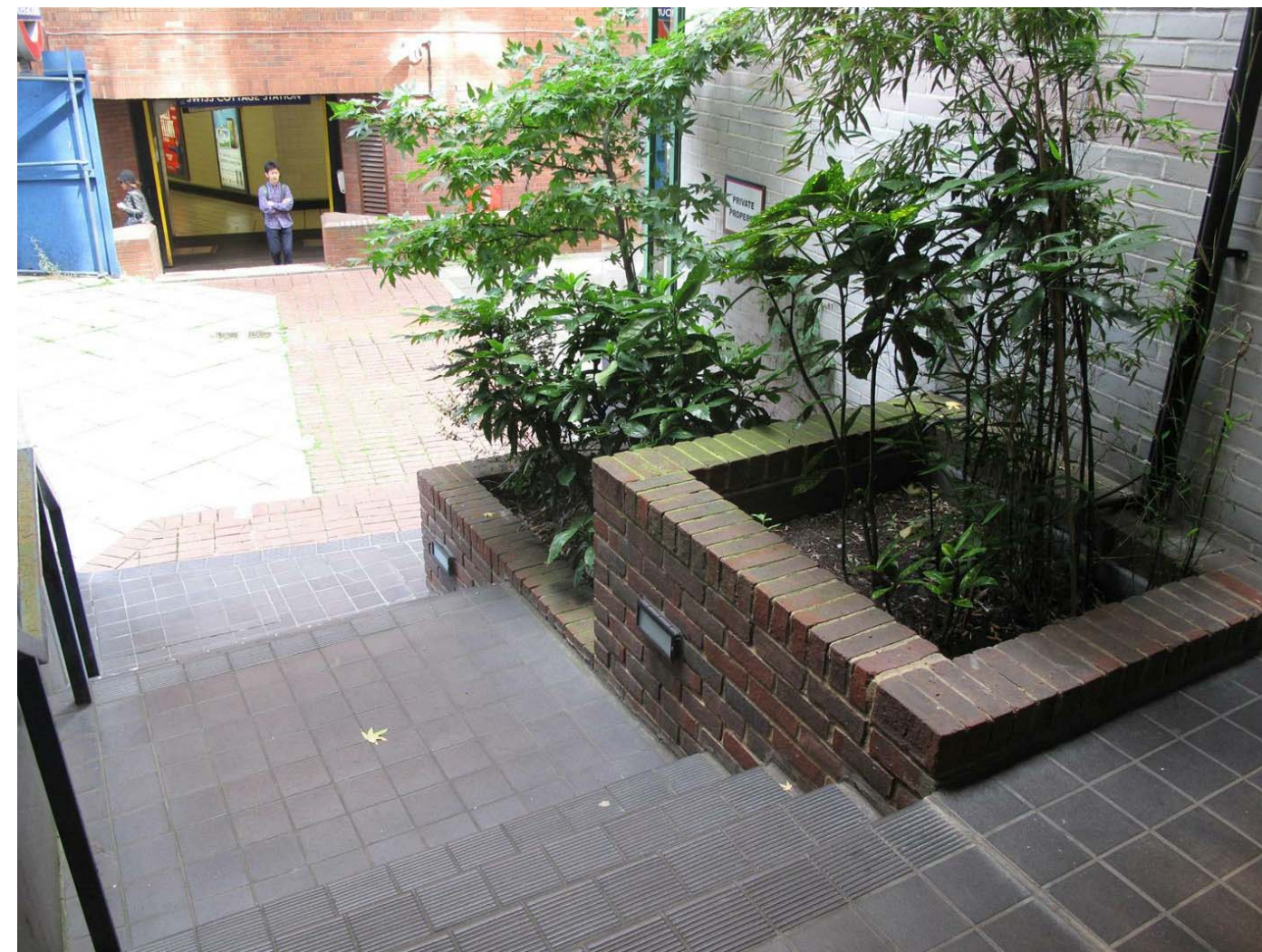
6 Existing handrail, floor tiles and brick planters
