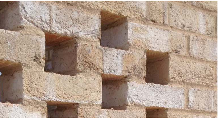
Figure 1: Indicative Brick Types; (from the top) buff (to clad the darker 'skin' of the facade); white (to clad the lighter 'carved' areas of the facade); and hit and miss brickwork.
