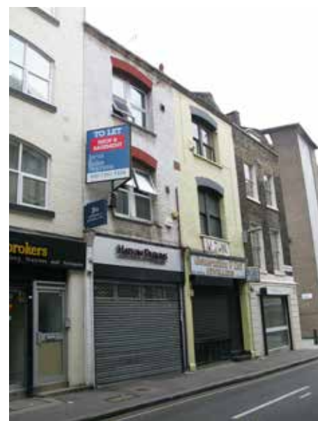
VIEW OF HATTON WALL FACADE LOOKING EAST
