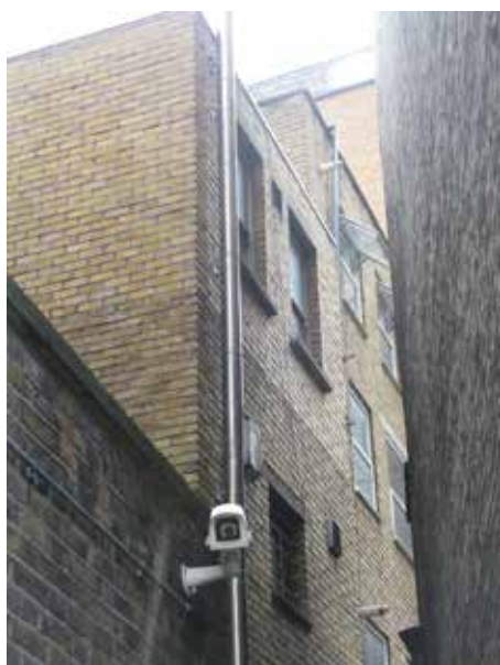
VIEW OF REAR FACADE LOOKING WEST
