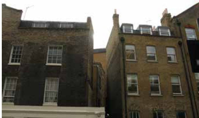
HATTON GARDEN Mansards & dormers are a consistent style for roof extension in the area
