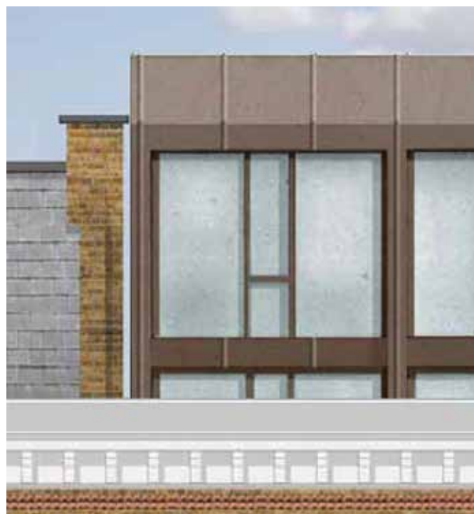
23-27 HATTON WALL Visualization of zinc clad roof extension set back behind parapet (under-construction)
