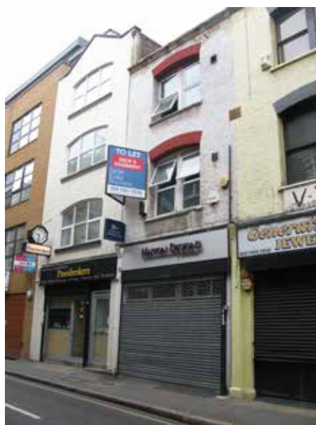
VIEW OF HATTON WALL FACADE LOOKING WEST
