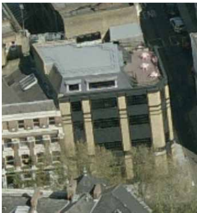
154 CERKENWELL ROAD Zinc-clad mansard roof with dormers and roof terrace
