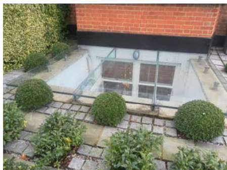
(3) Light well, No. 16 Kidderpore Gardens - View 1
