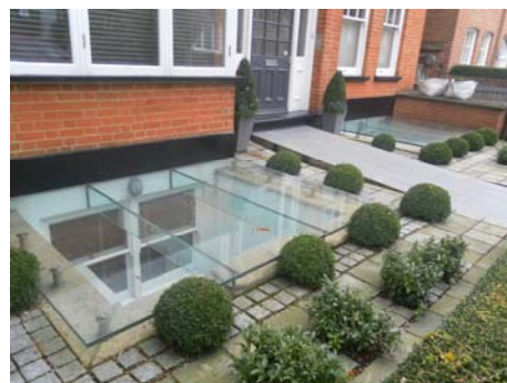
(4) Light well, No. 16 Kidderpore Gardens - View 2
