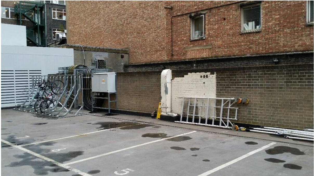
View of proposed site for new plant with commercial property façade in background – looking north
