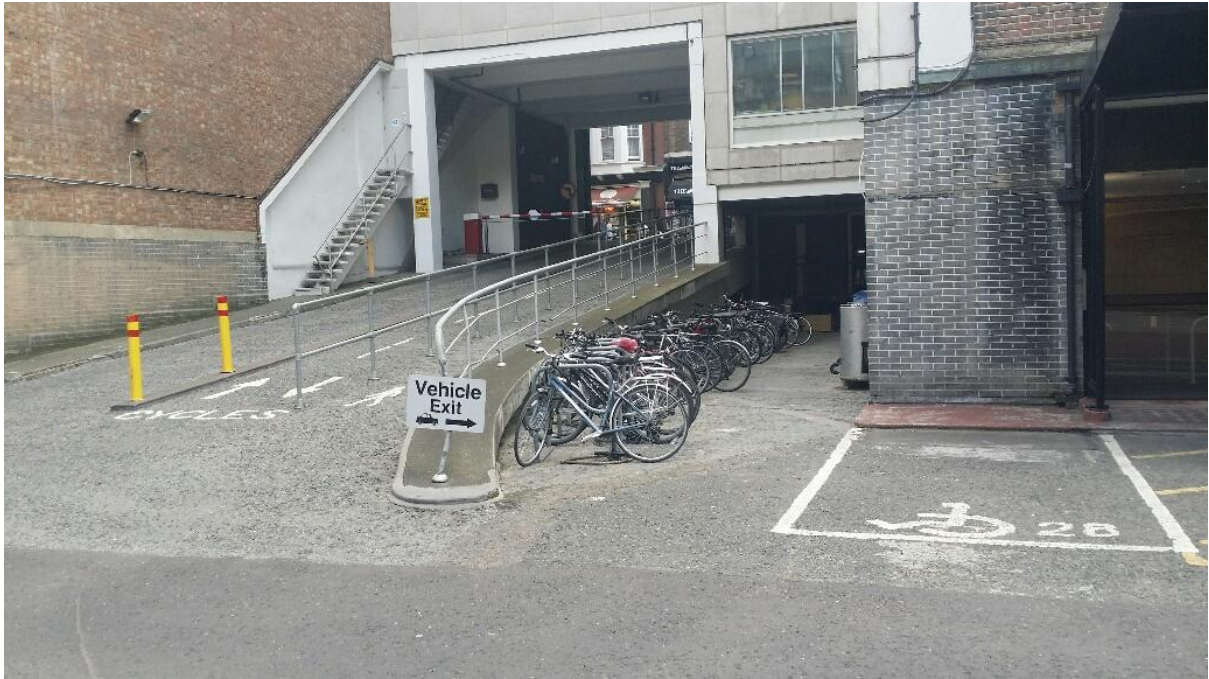
View of ramp to street level – looking south
