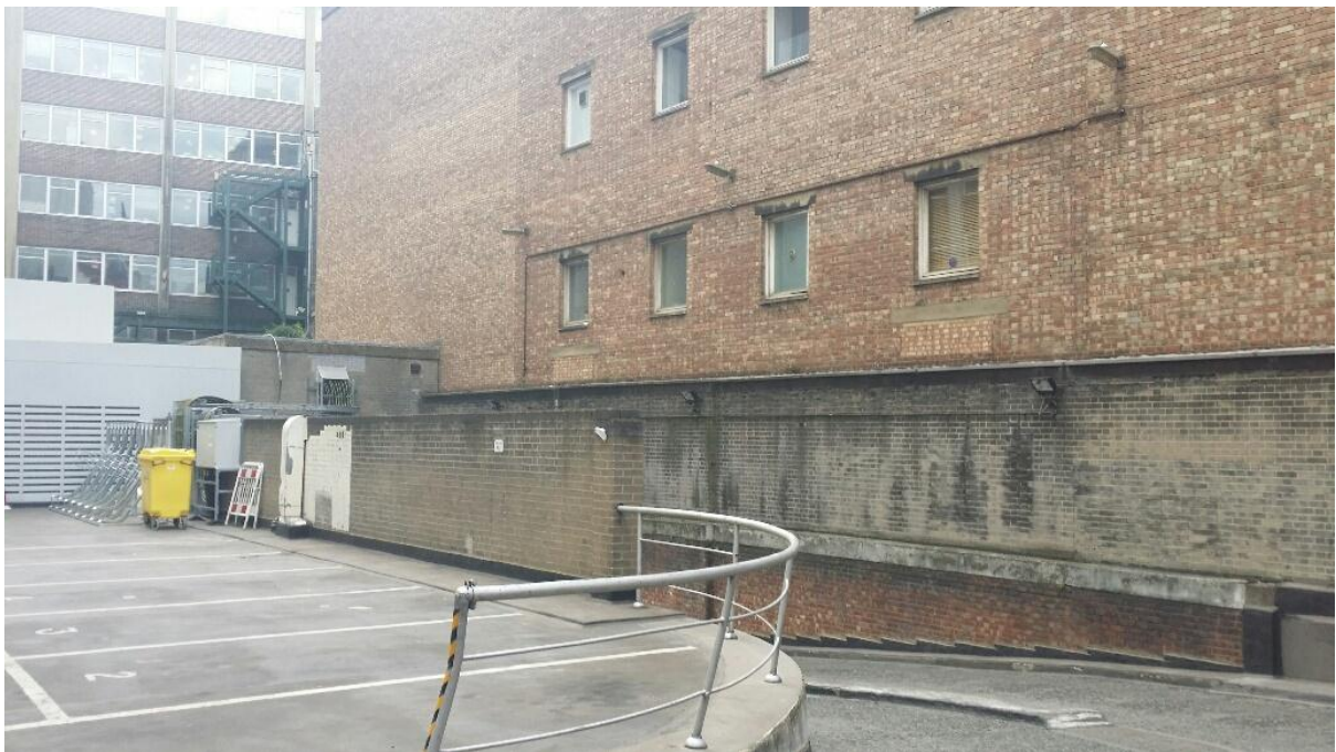
View of down ramp to car park – looking north
