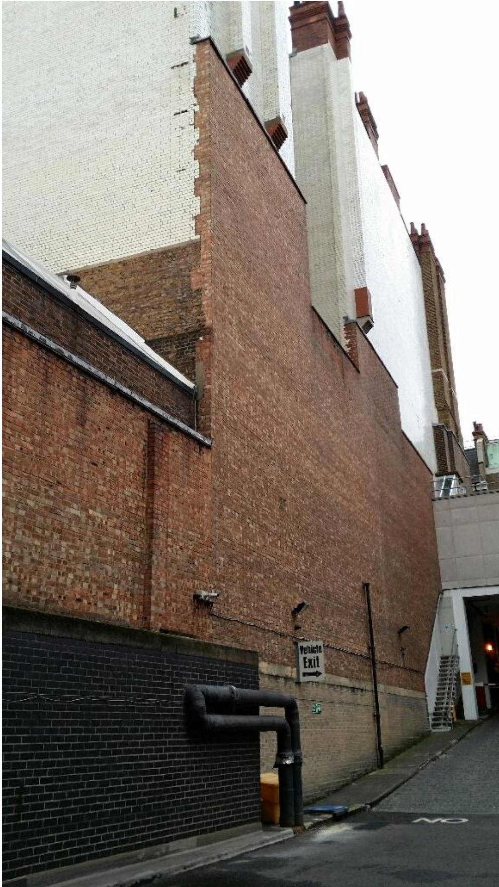
View of nearest noise sensitive property façade – looking south
