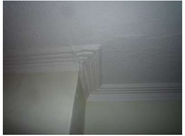
Fig 50 Cornice at front room, second floor
