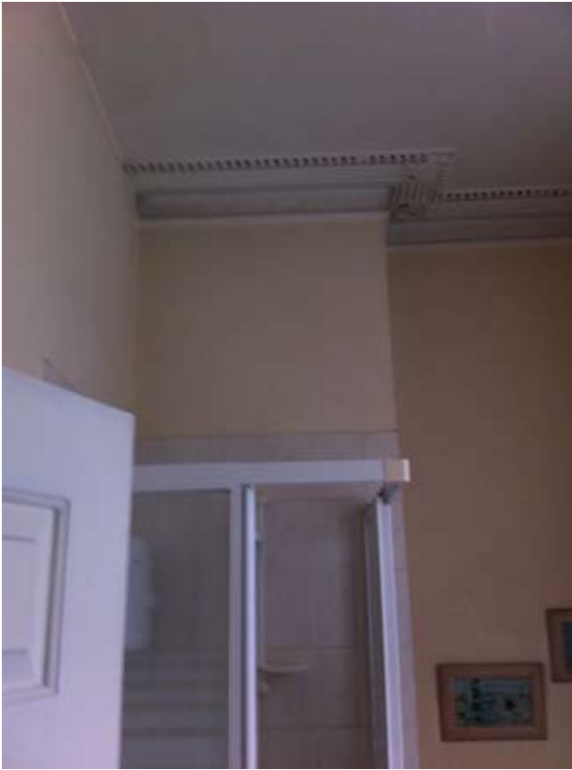
Fig 36 Bathroom within back room
