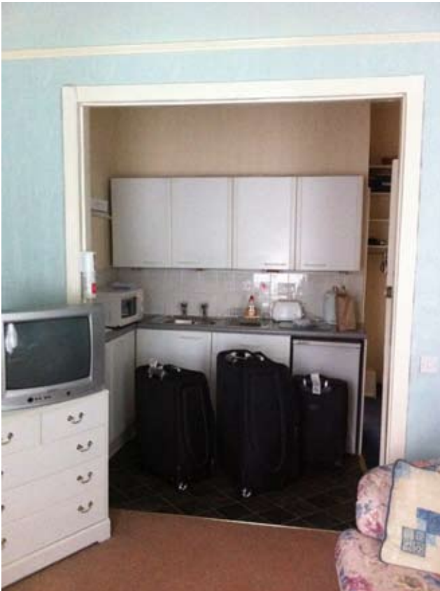
Fig 38 Kitchen opening through spine wall
