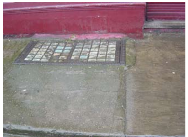
Fig 7 Pavement light to front lightwell
