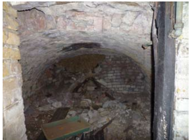
Fig 24 Left hand vault
