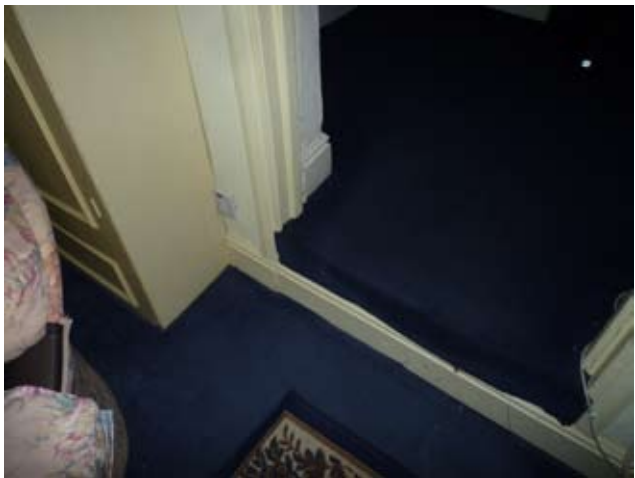
Fig 45 Step up between back room and infill
