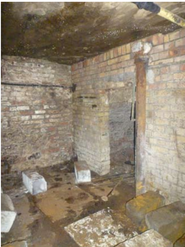
Fig 22 Front lightwell with concrete roof covering
