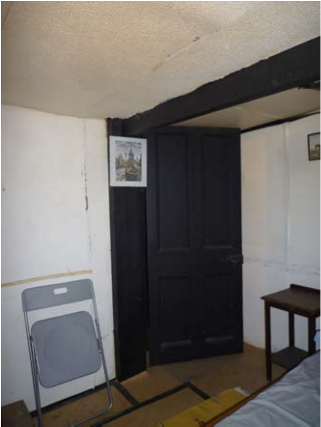
Fig 29 Basement space below main building
