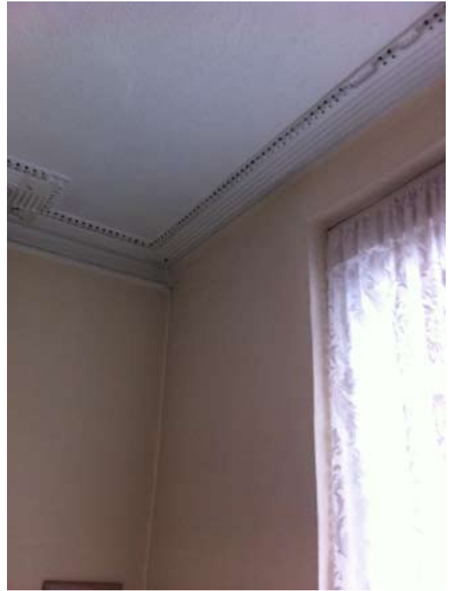
Fig 37 Bathroom within back room
