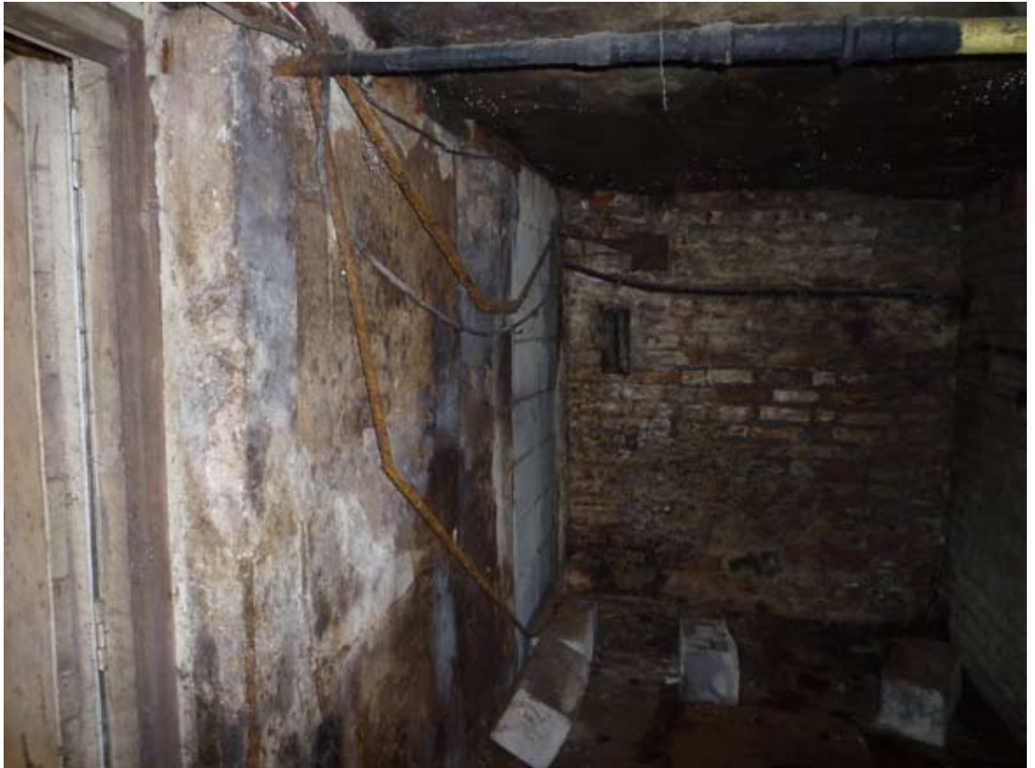
Fig 21 Basement front lightwell with concrete roof covering
