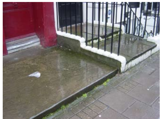
Fig 6 Concrete covering to front lightwell
