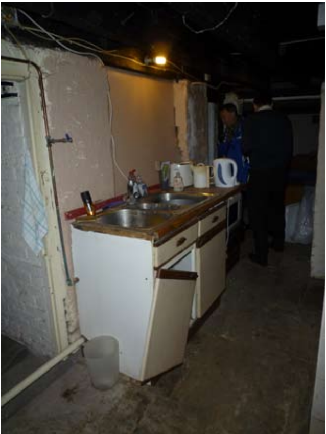
Fig 31 Basement corridor belwo ground floor infill
