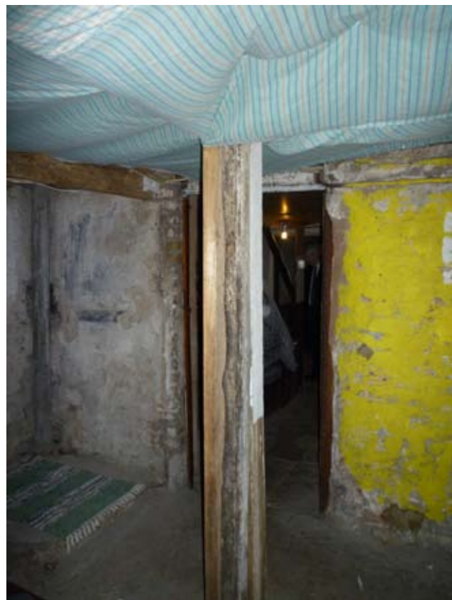
Fig 26 Basement space below ground floor infill
