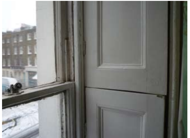
Fig 39 Timber shutter to front windows
