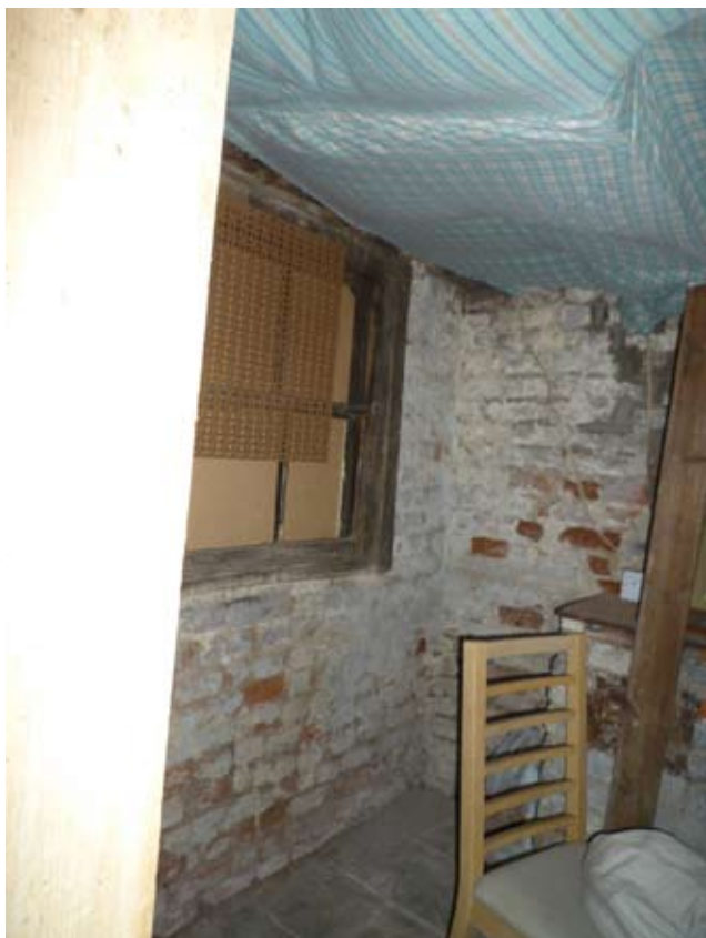
Fig 25 Basement space below ground floor infill
