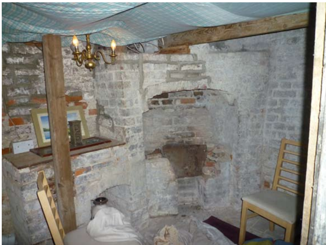
Fig 27 Basement space below ground floor infill
