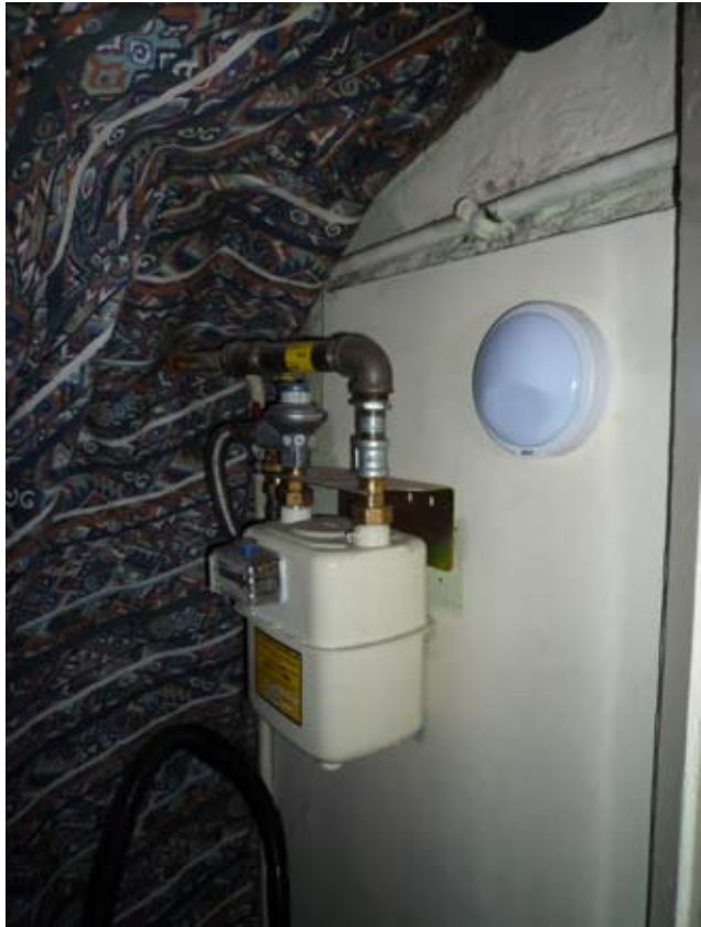
Fig 54 Below stair cupboard at second floor
