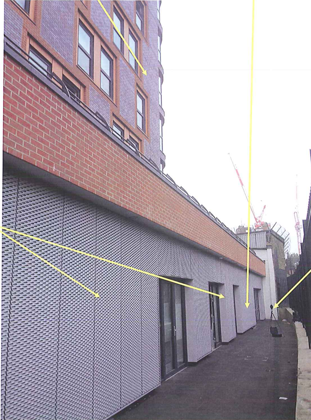
PHOTO B: Position of microphone and proposed location of air cooled condensers.
