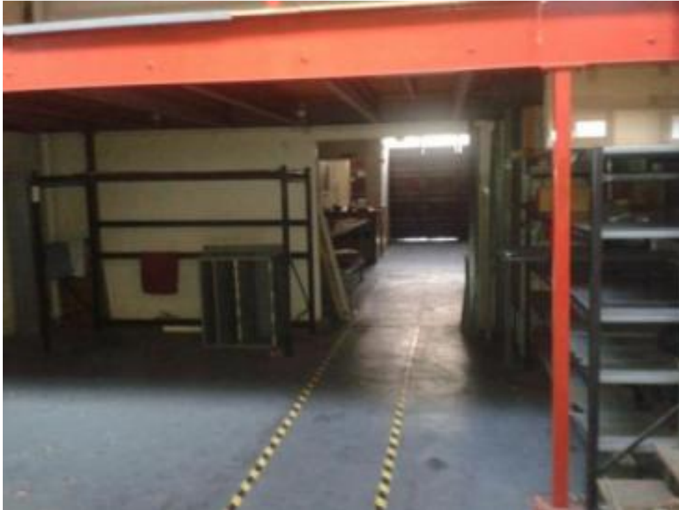
Photo 03: Internal View of Extension
