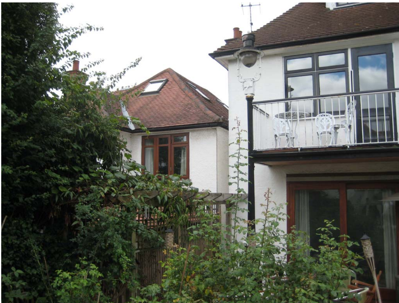
FIG 2 VIEW OF OLD BALCONY/TERRACE TOWARDS NEIGHBOURING PROPERTY
