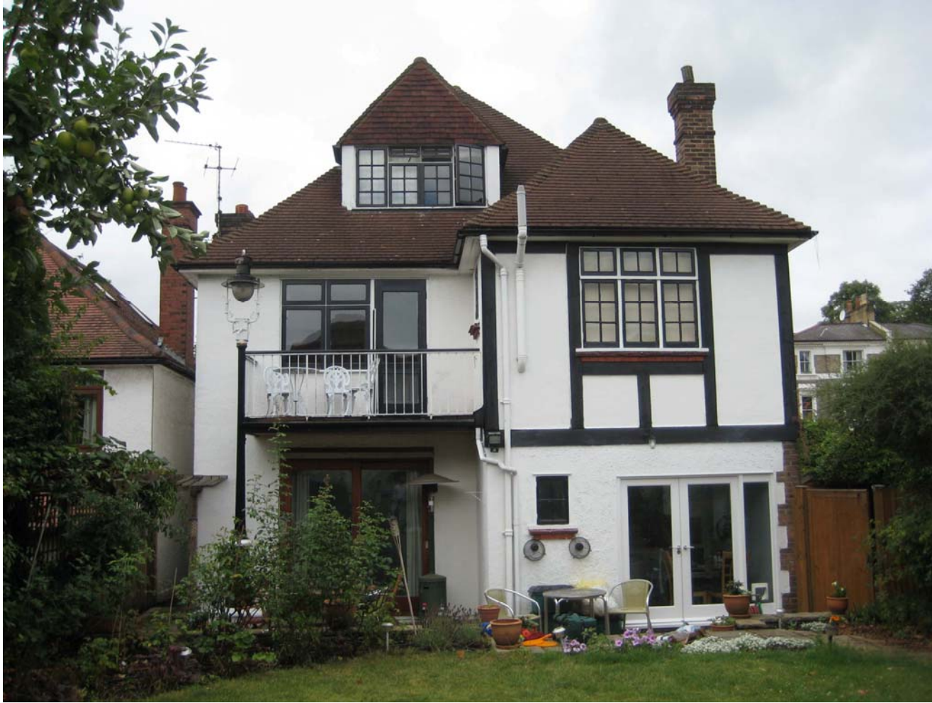
FIG 1 OLD FIRST FLOOR BALCONY/TERRACE TO REAR REMOVED (2013) TO ALLOW FOR NEW REAR EXTENSION
