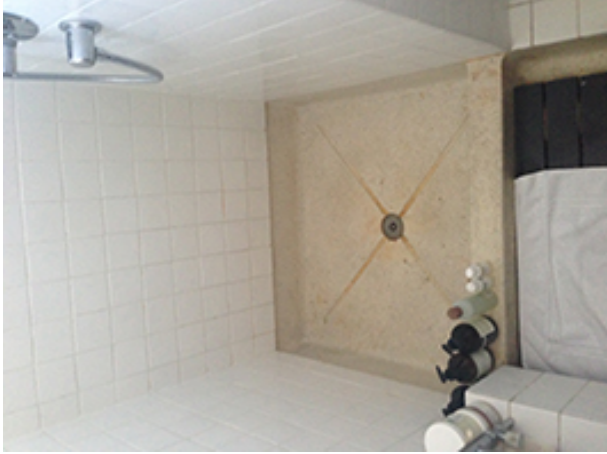
3. Existing Shower room detail
