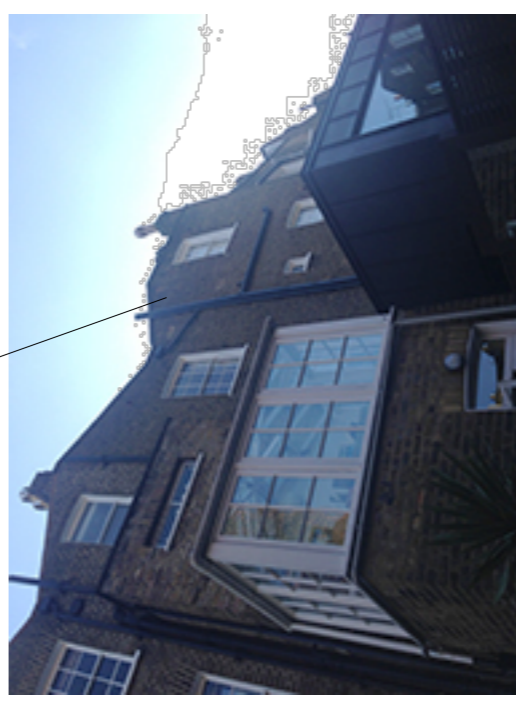
4. View to No.35 Rear Elevation
