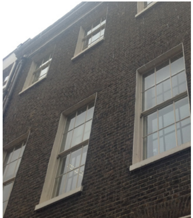
The existing sash windows are to be sensitively restored and their thermal and acoustic performance upgraded.
