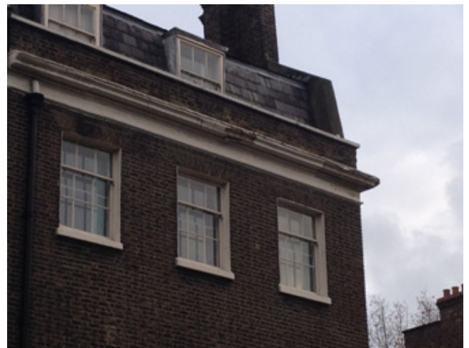
Essential maintenance work to the external envelope is required including repair of the cornice and renewal of the existing lead flashing.
