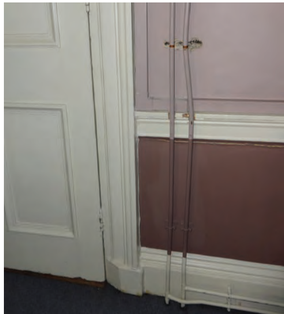
Visually intrusive surface-mounted services
