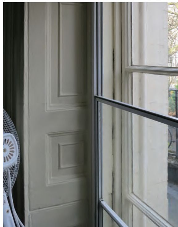
Unsympathetic secondary glazing prevent opening of shutters
