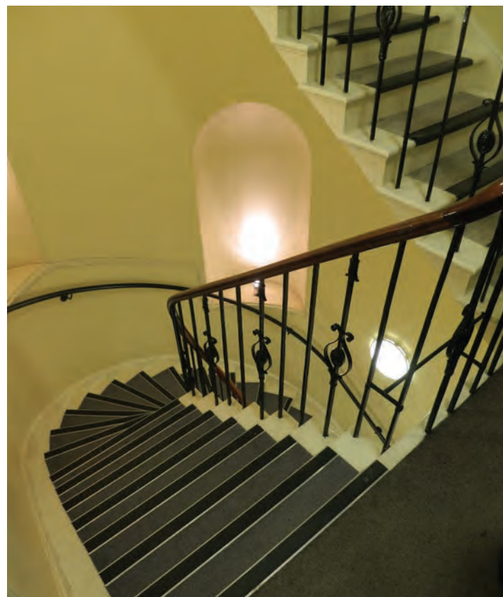
The staircase, with its daring cantilever steps and slender wrought iron handrail, is the most impressive feature of 11 Bedford Square. The wall-fixed handrail was added after 1968, and the carpet treads and heavy nosings detract from its significance.
