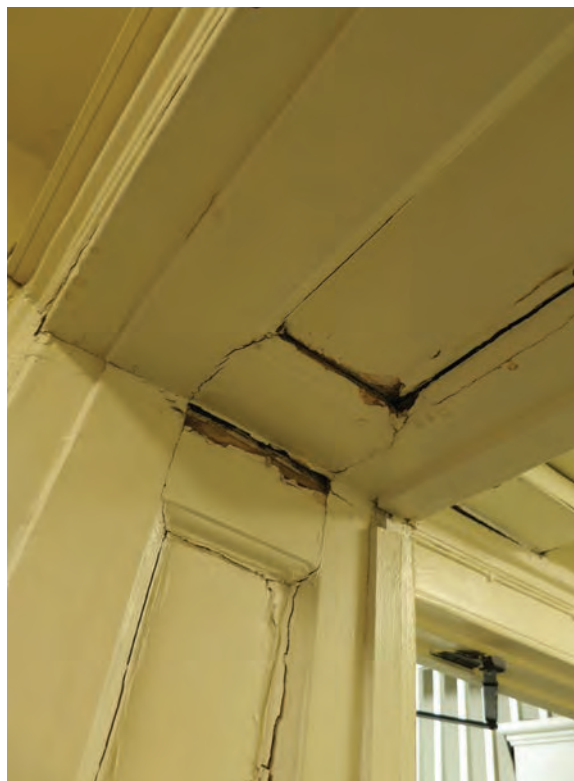
Water damage to joinery on third floor
