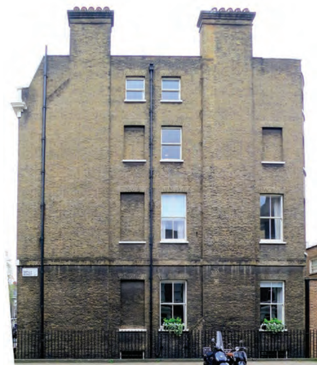
The side elevation of 28 Bedford Square, which is not visible from the square itself. As on the south elevation of no.11, the elevation has a regular pattern of window-sized bays, with a fairly random arrangement of actual windows.
