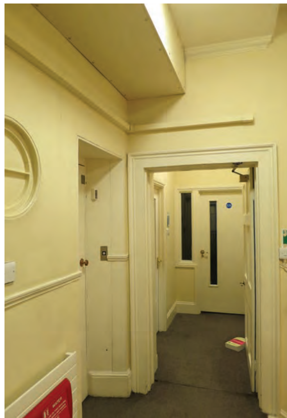
Unsympathetic modern boxing, trunking, fire doors and partitions
