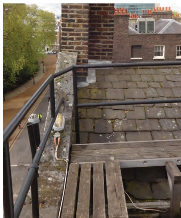
Obsolete fire escape over the roof
