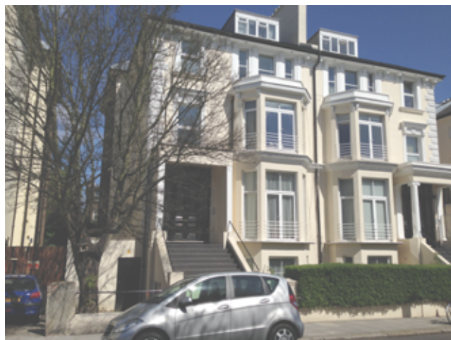
Adjacent terrace 9-15 Lancaster Grove
