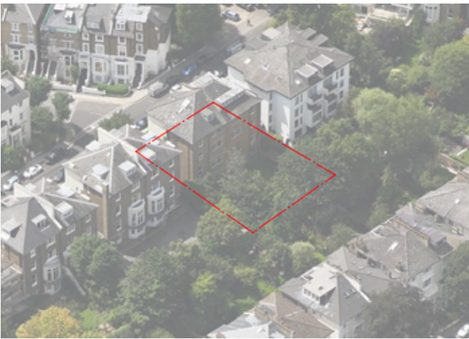
Aerial view of site from north-east
