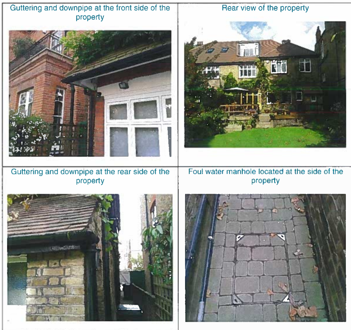
Figure 2 – Existing building on development site
