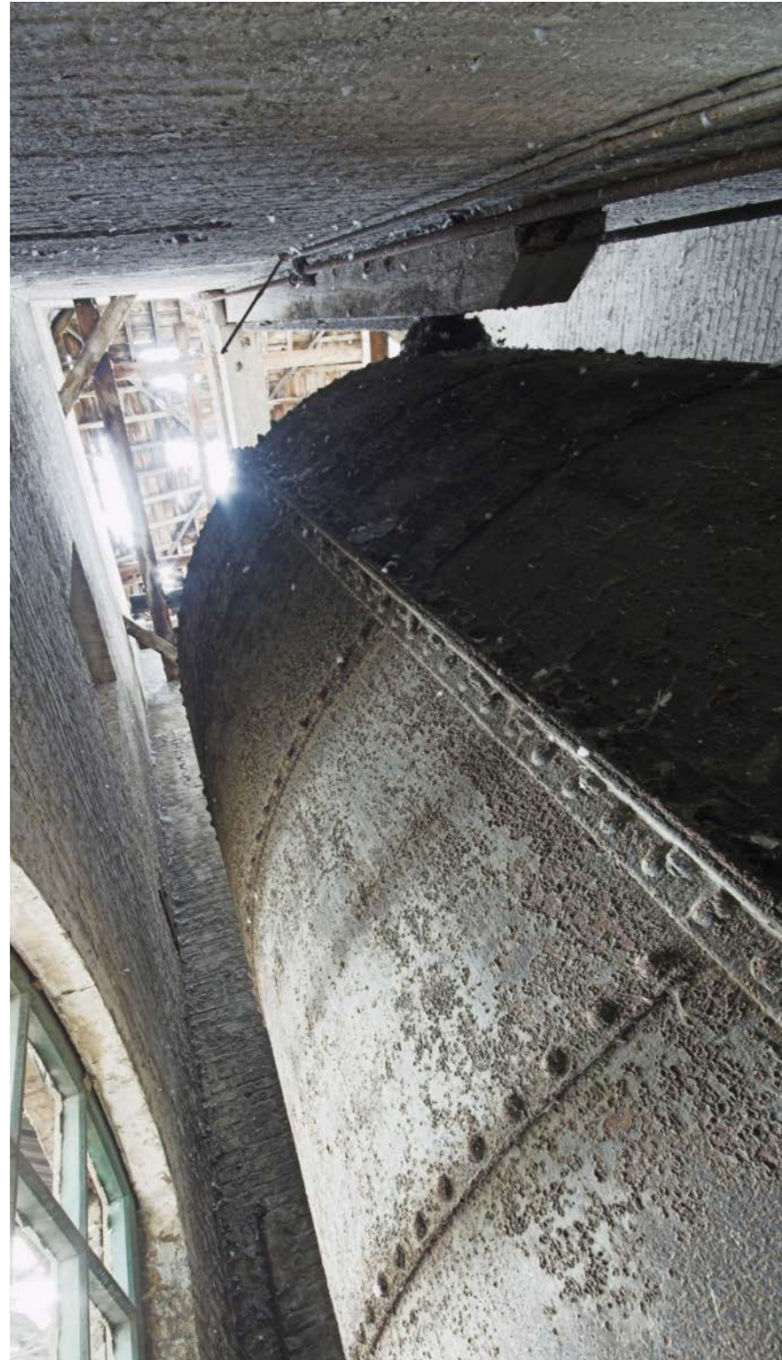
Accumulator Tower - Interior view of weight case
