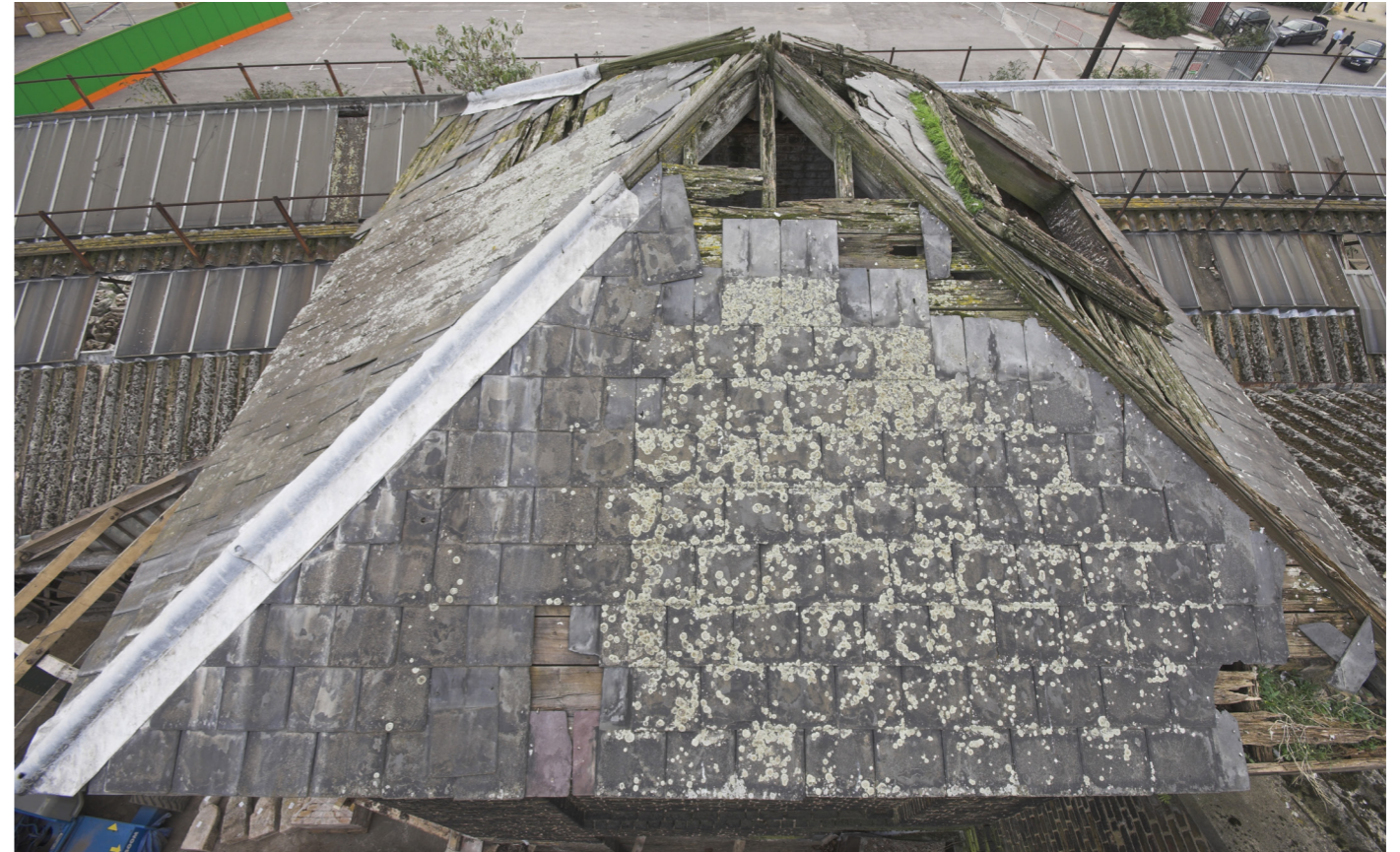
Condition of existing accumulator tower roof
