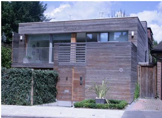
Street View of the Camden Passivhaus
