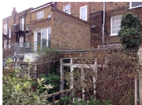
03 – Neighboring rear extensions (no 13 & 15)
