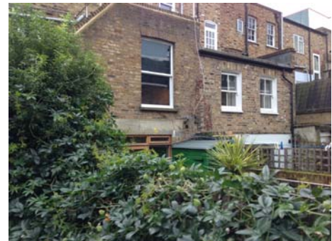
04 – Neighboring rear extensions (no 13 & 15)
