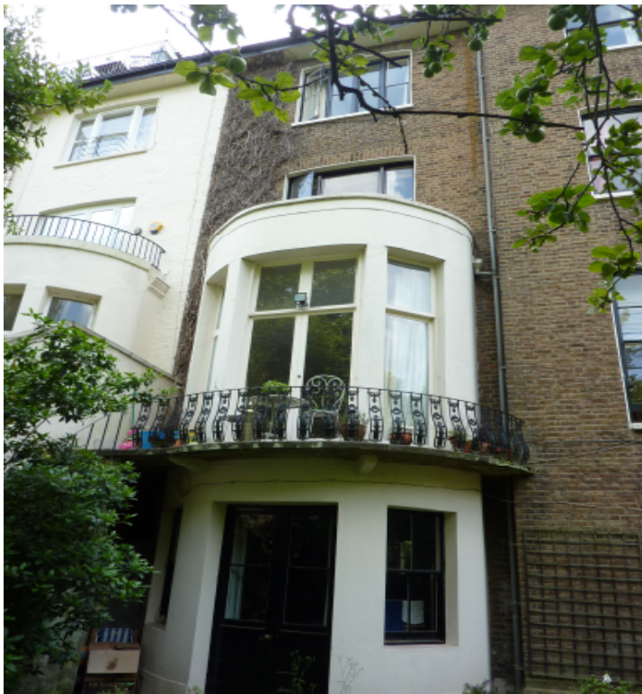
2. Rear elevation showing existing bay and neighbours railings at second floor level
