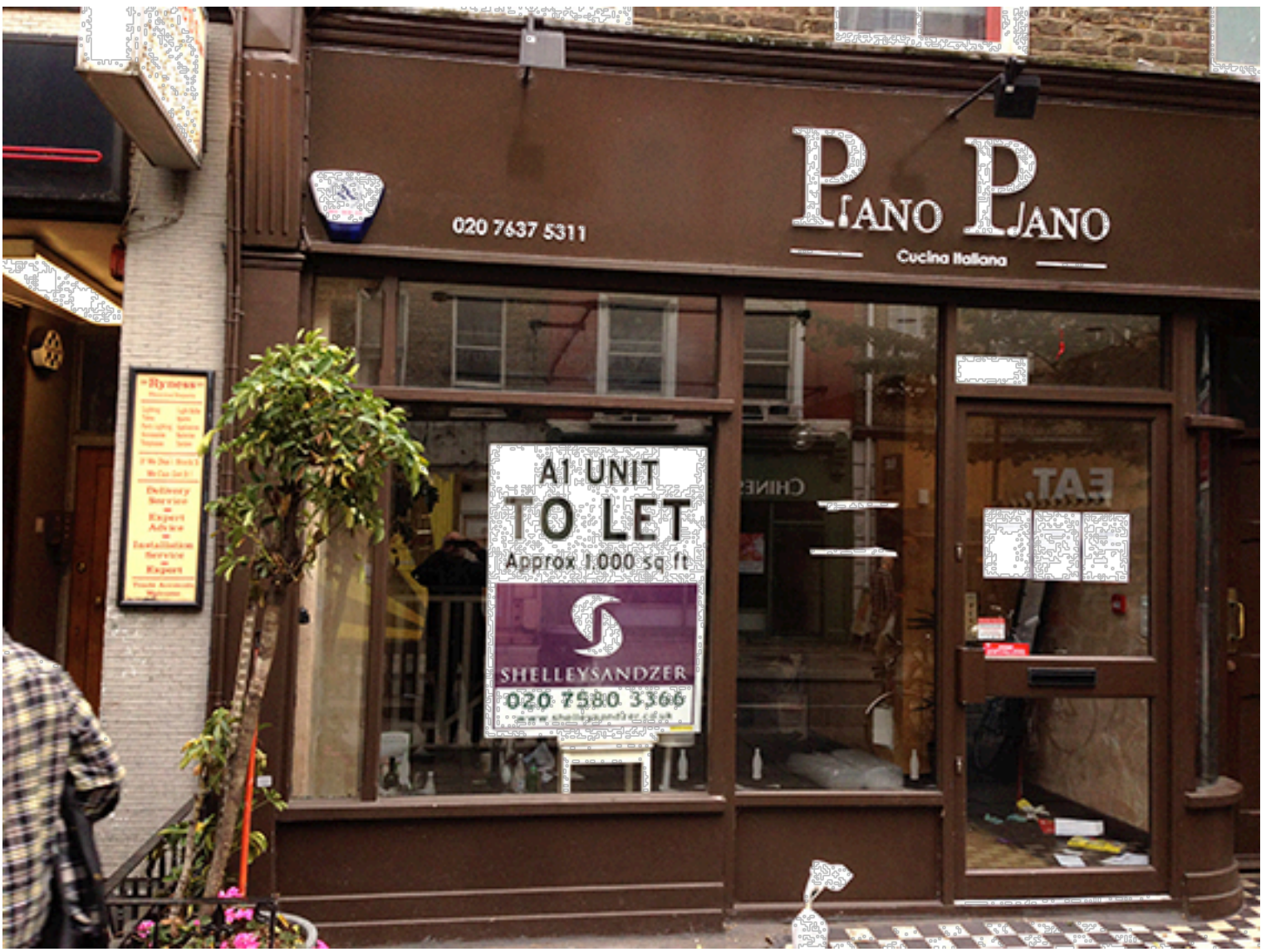
THE ABOVE IMAGE SHOWS SHOPFRONT AS EXISTING WITH PART TIMBER/PART ALUMINIUM ARRANGEMENT
