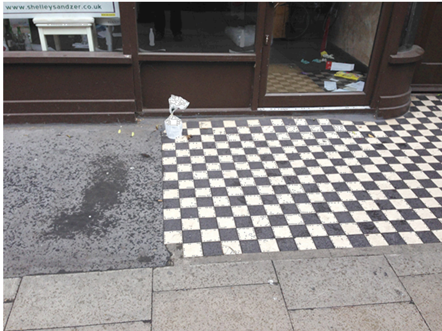
THE ABOVE IMAGE SHOWS TILING AS EXISTING WITH PART BITUMEN COVERING
