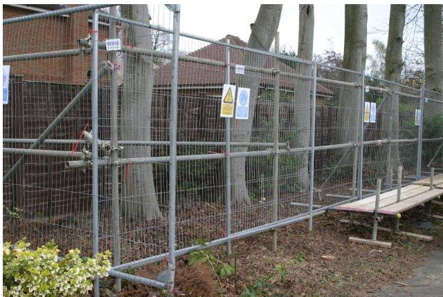
Scaffolding within the RPA Avoiding Crown and Stem Damage
