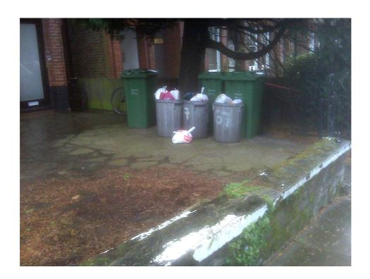
The paved yard is cracking up and the boundary wall is bellied towards the pavement.
