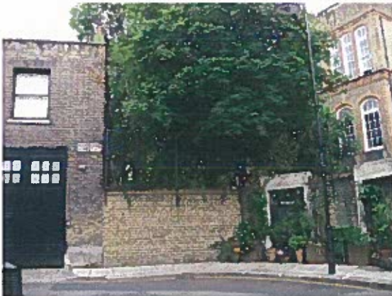
3. Section of wall to be re-built.
