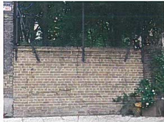
4. Close-up of section of wall to be re-built.
