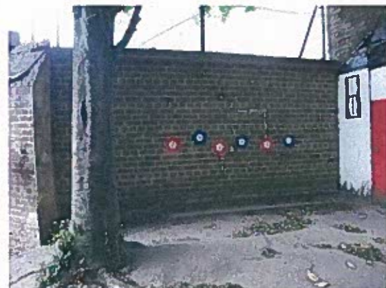
6. Close-up view of wall from inside of School.
