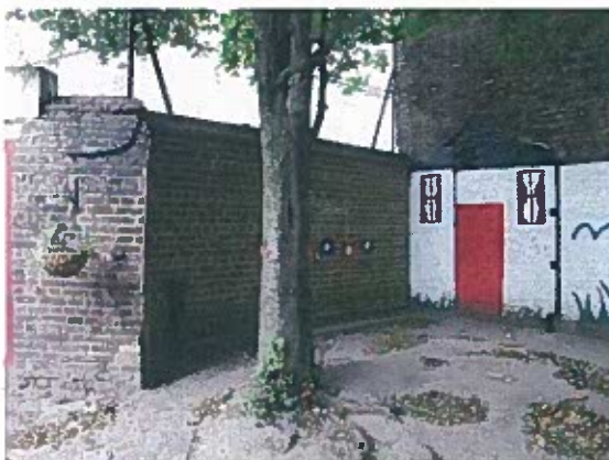
5. View of wall from inside of School.
