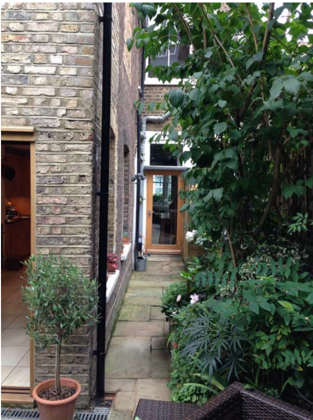
Figure 2 - View of rear where the infill extension is to be located
