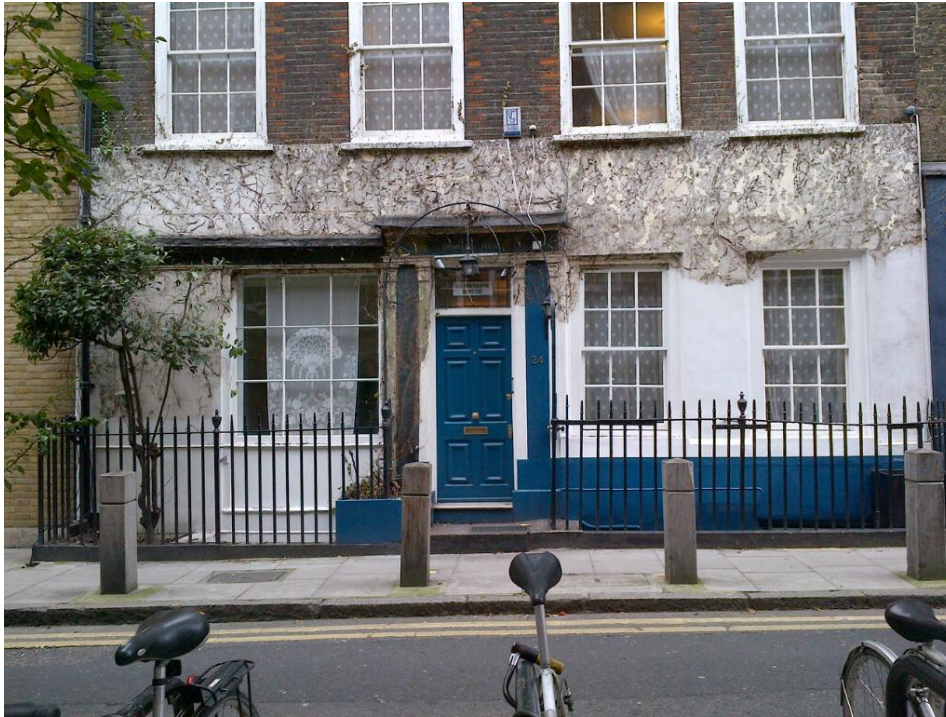
Figure 5: 24 Betterton Street entrance door
