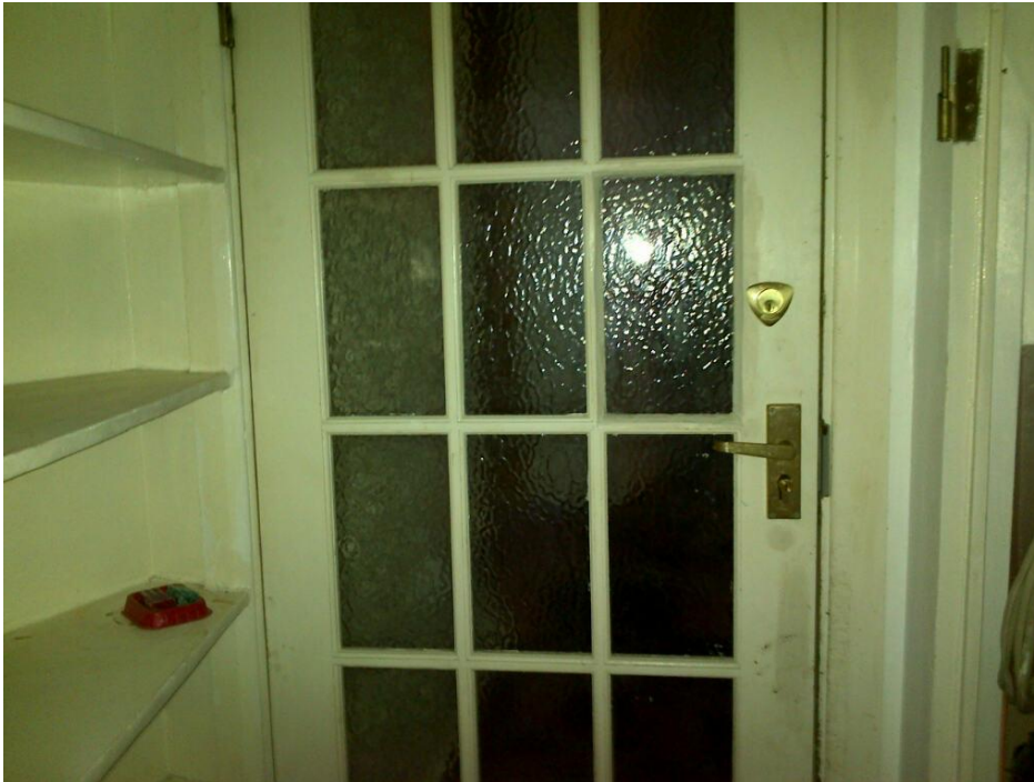
Figure 4: Yale locked door viewed from Basement Flat (Lower Ground, 24 Betterton Street)
