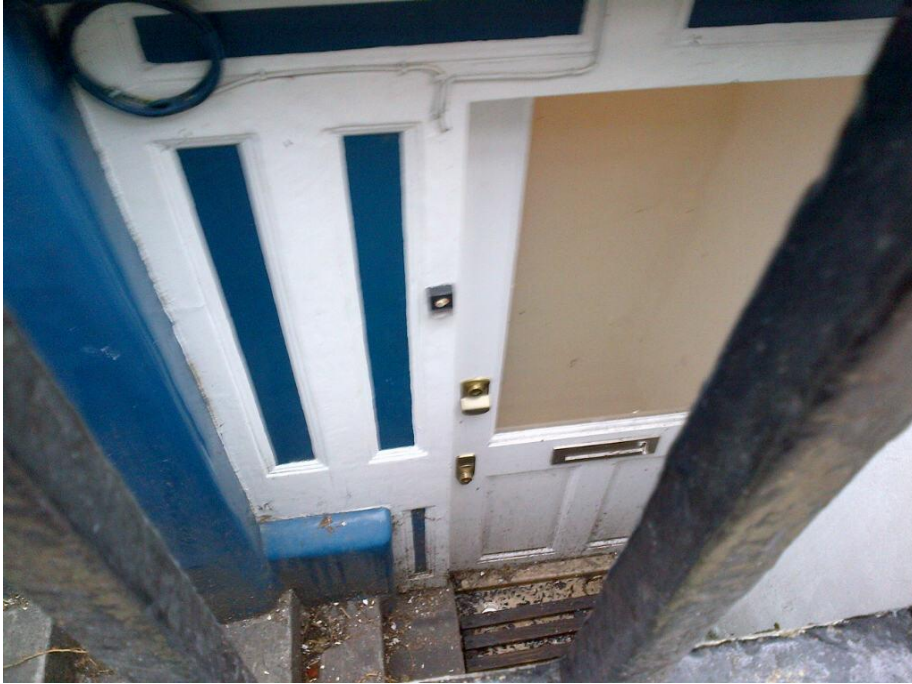
Figure 2: Basement Flat entrance door
